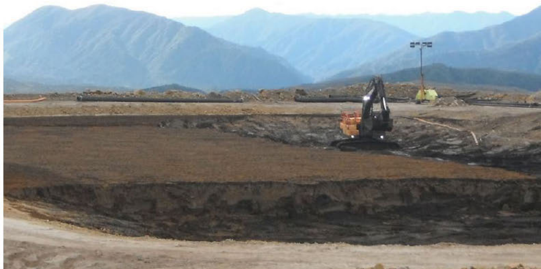
Figure 6. Mangatini Filter Bed #2 cleaning in progress July 2024
