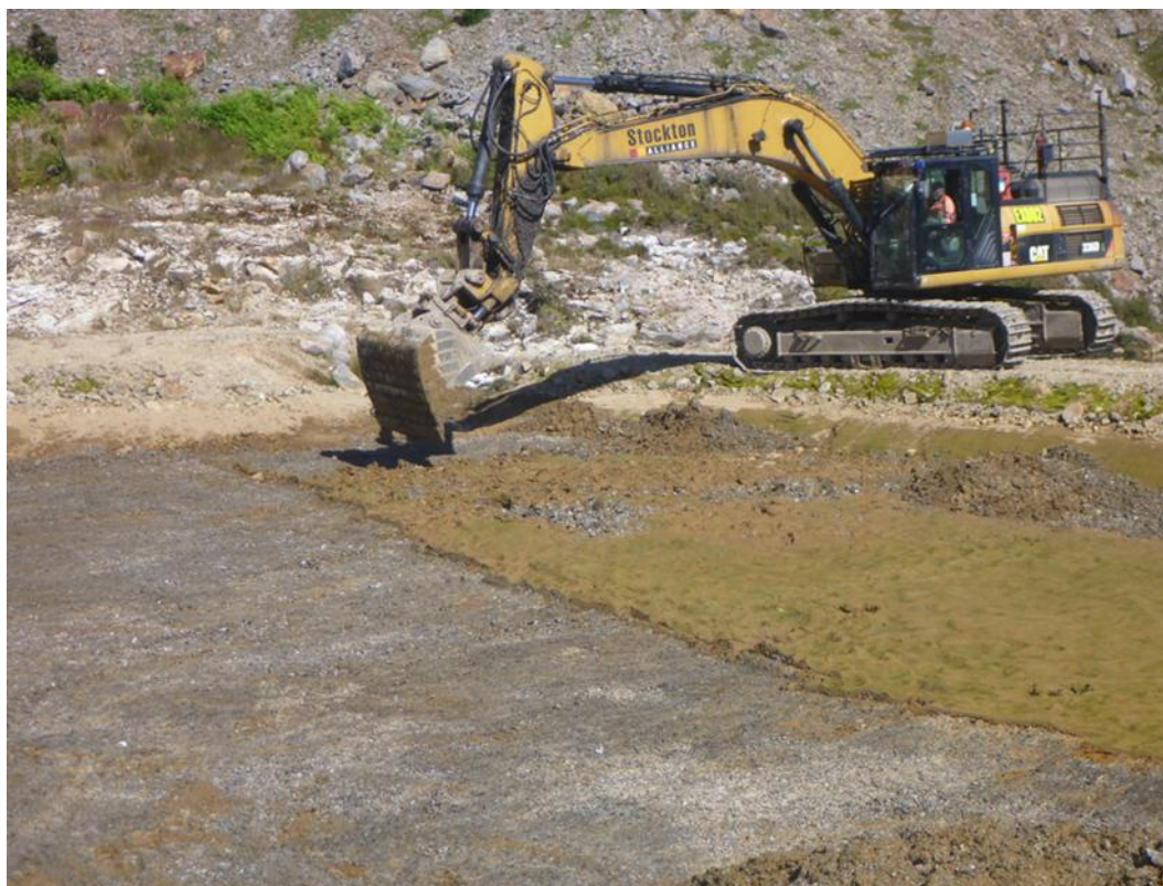
Figure 13. Clean out of Whirlwind MSR AMD passive treatment system sludge, 2025
