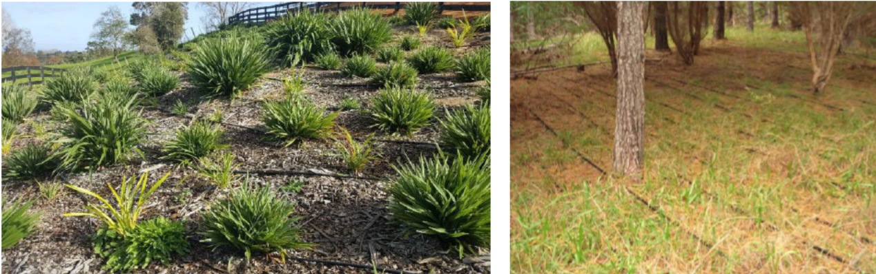
Figure 13- Examples of Installation of surface laid drip irrigation fields
