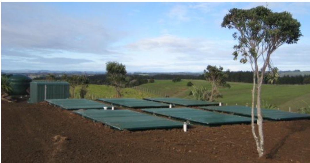
Figure 10- Example of AX100 installation
