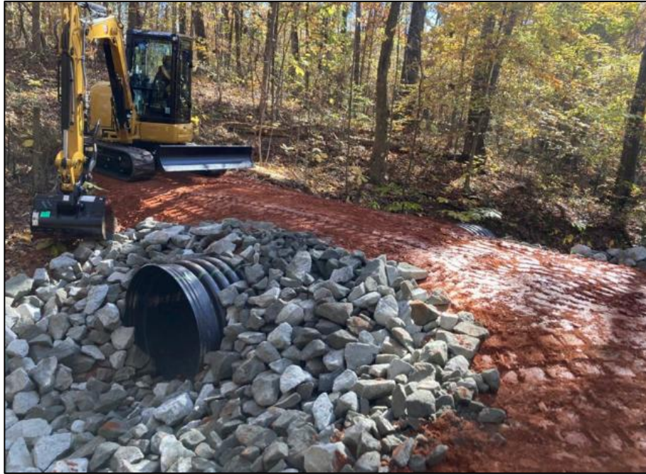
Figure 3-26: Culvert example (Stantec, 2026d).
