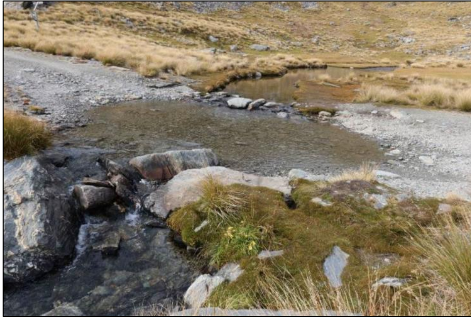
Figure 3-25: Splash crossing (ford) example (Stantec, 2026d).
