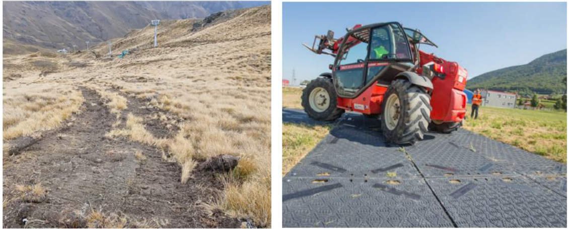
Figure 3-27: Example of temporary access track (left), rubber matting for use near critical source areas (right).
