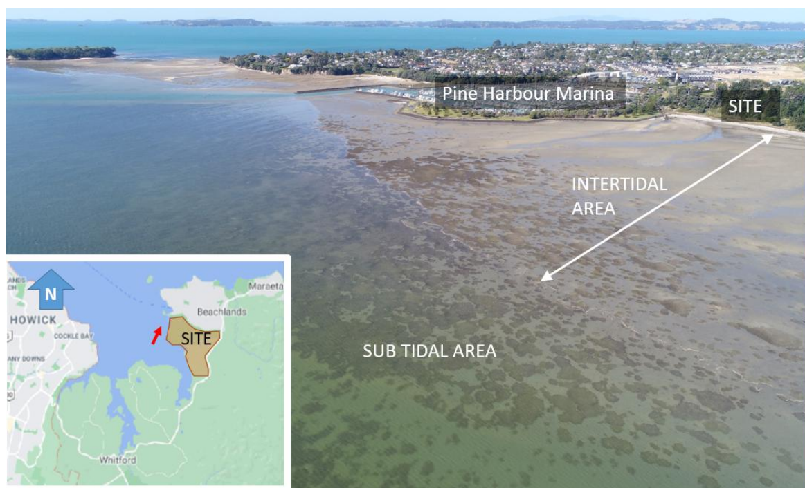
Figure 3.2: Looking towards northern extent of site.
