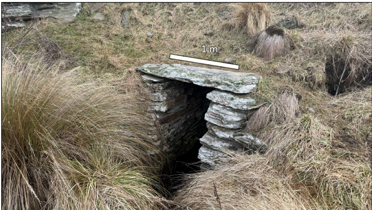
Figure 240. View of Culvert intake.
