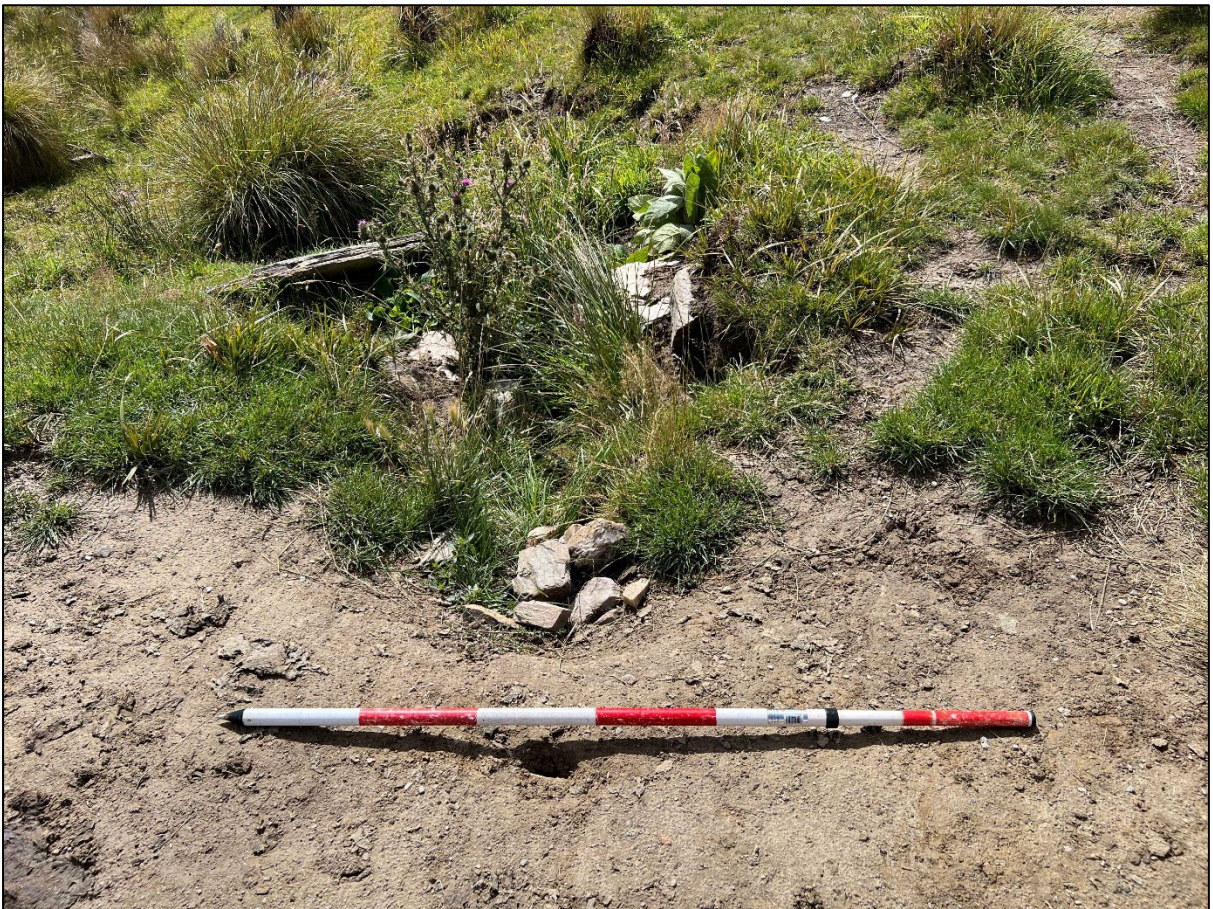
Figure 233. Stone-lined dam outlet, looking north-east.
