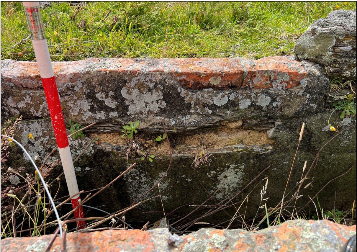
Figure 231. Detail of sheep dip showing mortared stone construction and brick top course.
