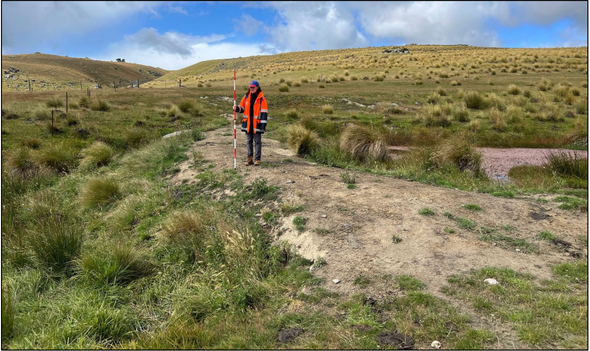
Figure 232. Dam, looking south-east.
