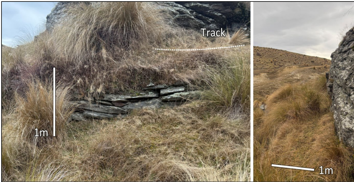
Figure 246. Left: View of revetting on section of I42/258 south of second outcrop (facing north). Right: View to west of track above revetting.
