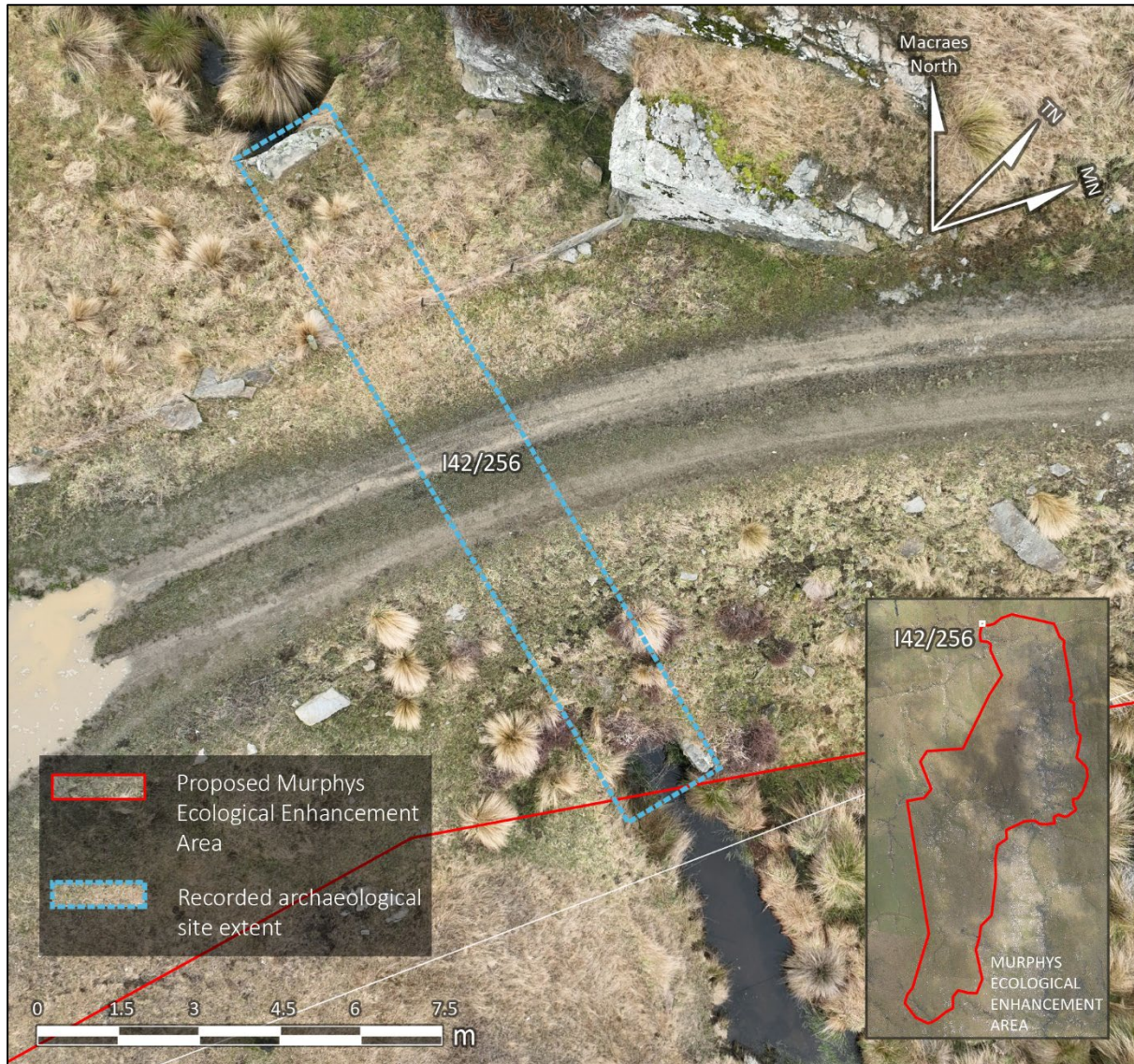
Figure 238. Aerial view showing location of Stone Culvert I42/256 (2025 OGNZL aerial photograph).
