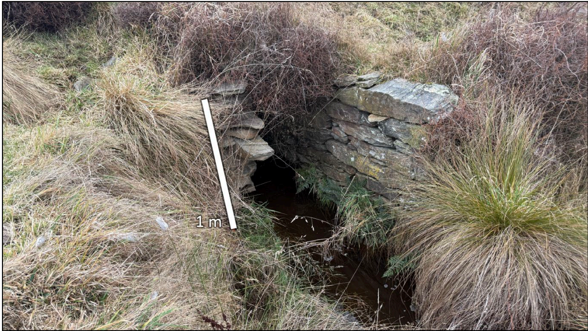
Figure 239. View of culvert outlet.
