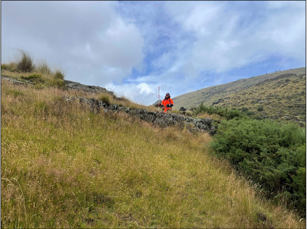
Figure 225. Stone revetment supporting the Ounce Battery water race (G) around the spur, looking south-east.
