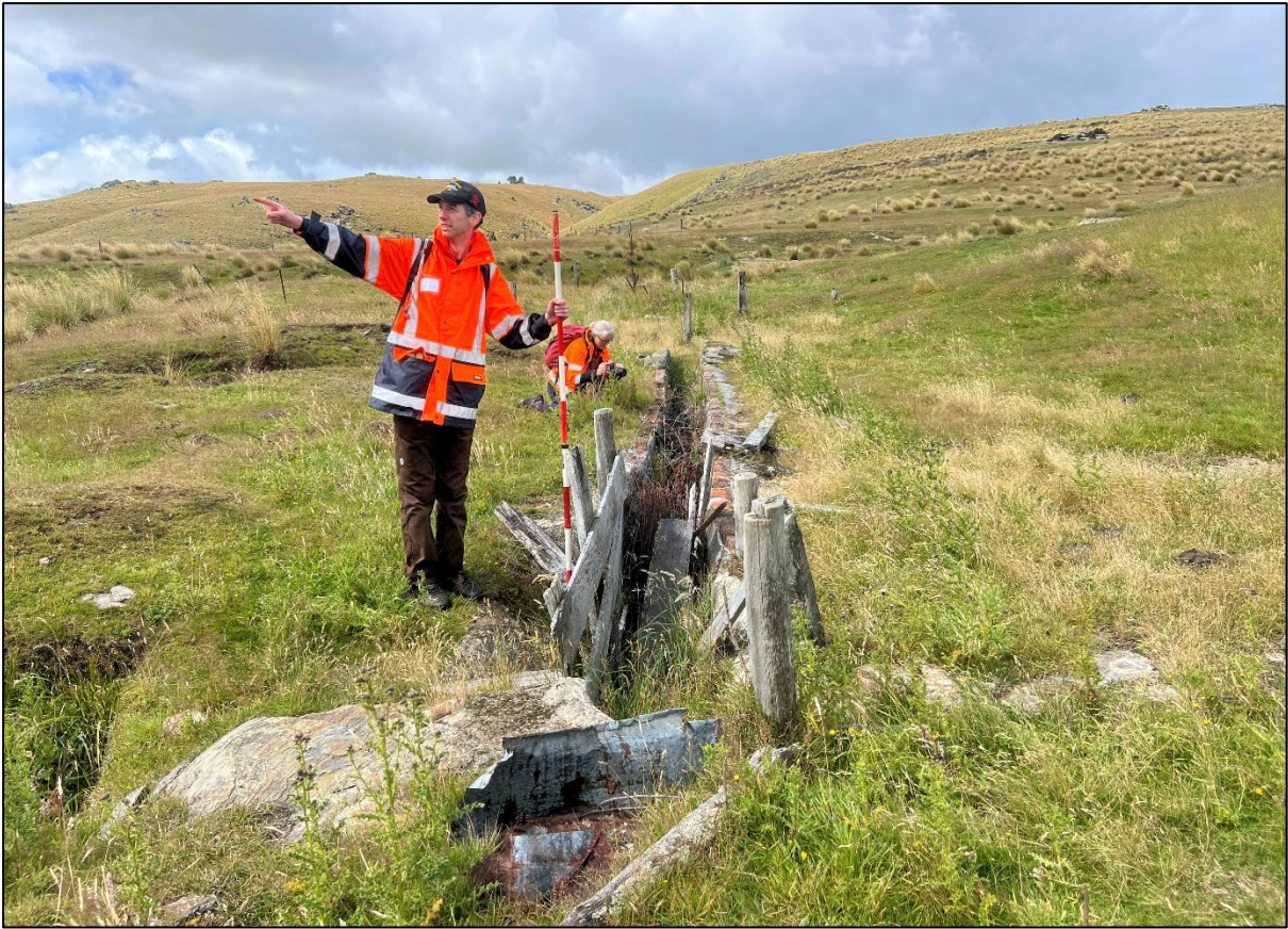
Figure 230. Sheep dip, looking south-east. Note exposed areas of paving at the lower right of the image.
