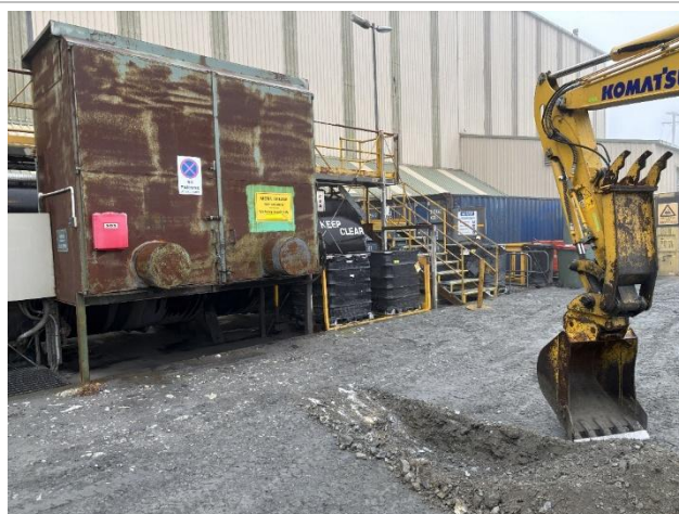
Photograph 2. Hydrocarbon storage - grease
