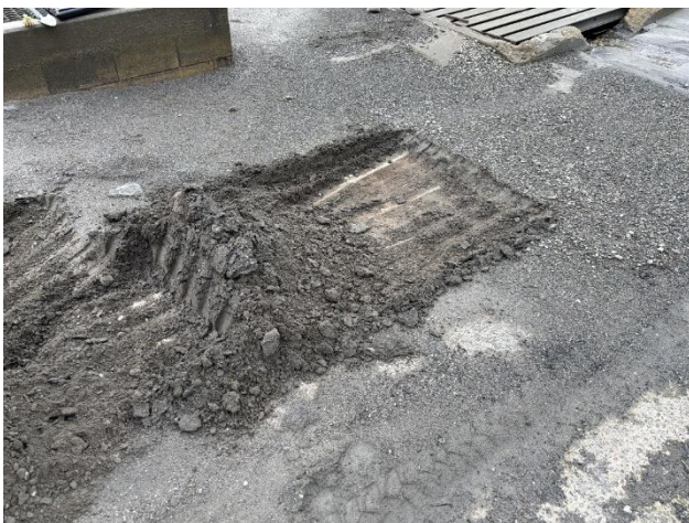
Photograph 17. Concrete identified beneath sediment at light vehicle wash bay
