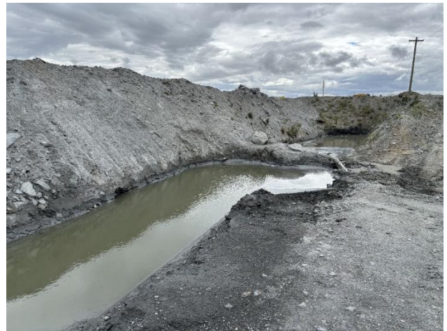
Photograph 14. First and second settling pond, separated by low bund
