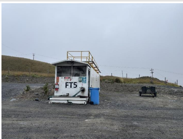
Photograph 27. Fuel farm looking south, raised ground visible to left and rear
