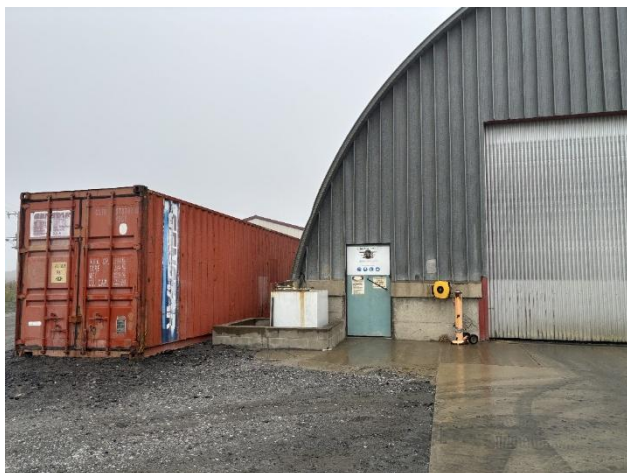
Photograph 9. Tyre workshop, showing concrete pad and small tank in bund
