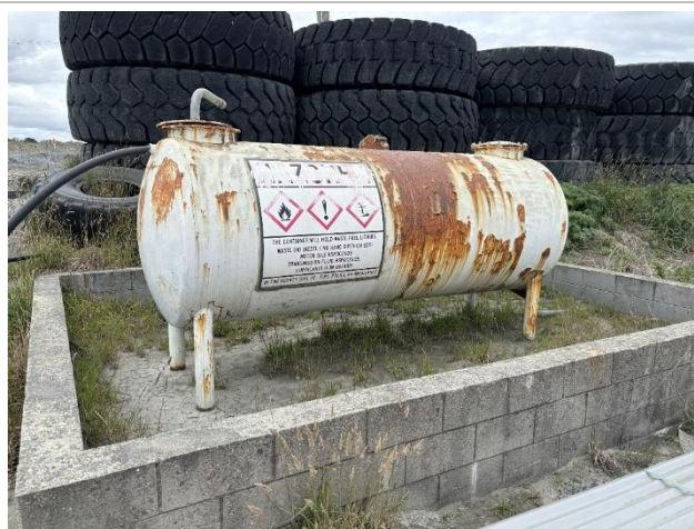
Photograph 22. Disused waste oil tank at southern laydown
