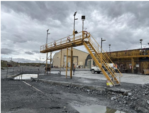
Photograph 13. Large vehicle wash bay. Concrete pad visible with scaffolding and containers. Water drains to the sump in the left of the image, and over concrete nib wall in centre of image
