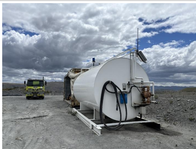
Photograph 20. Oil tank and northern laydown
