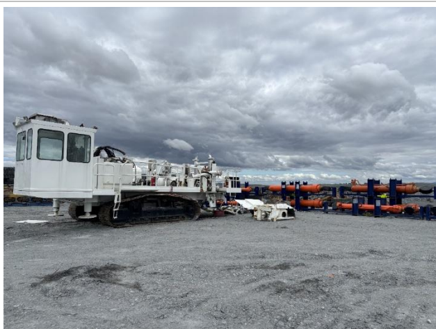
Photograph 19. Northern laydown area
