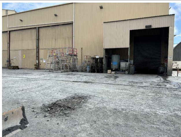
Photograph 4. Eastern side of workshop, slot drain discharges to the right of image
