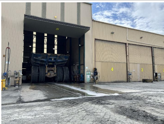
Photograph 3. Eastern side of workshop, wash water draining to slot drain
