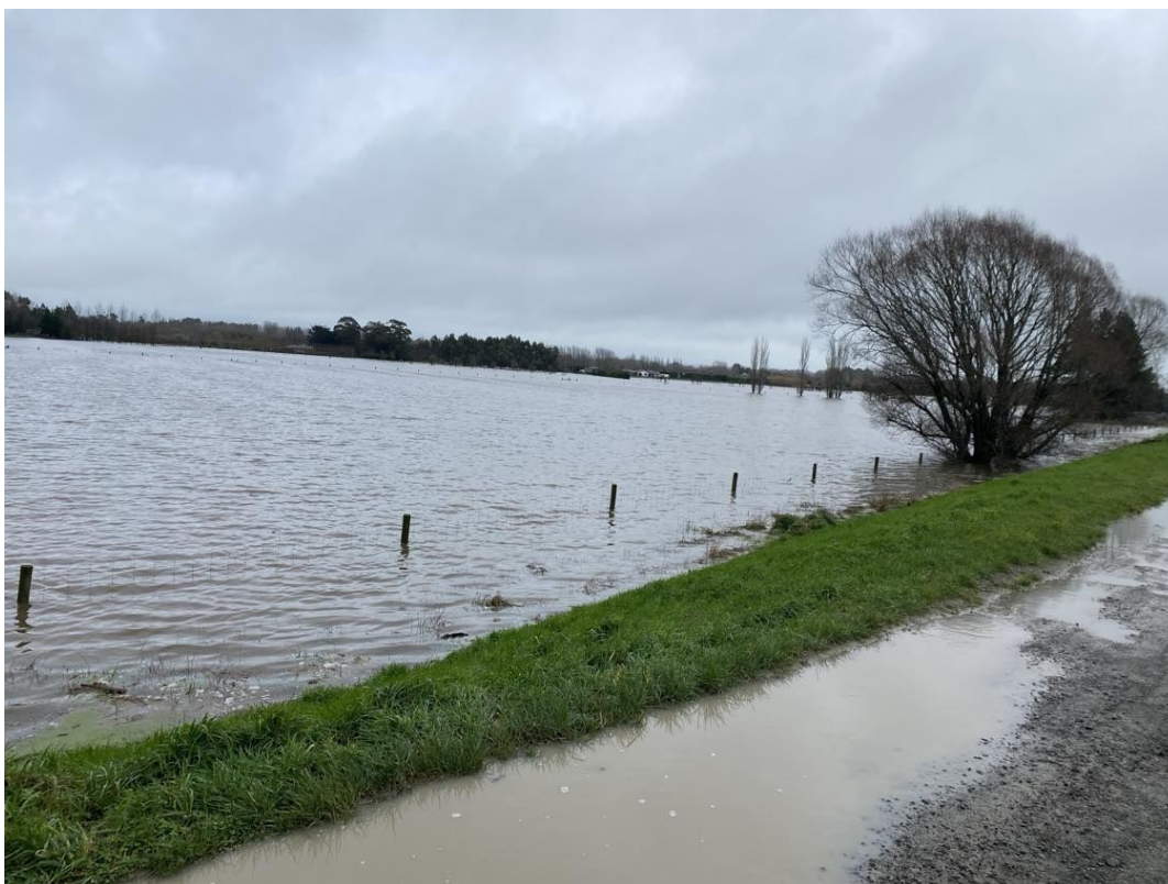
Figure 16: Threlkelds Road by the Cust Main Drain
