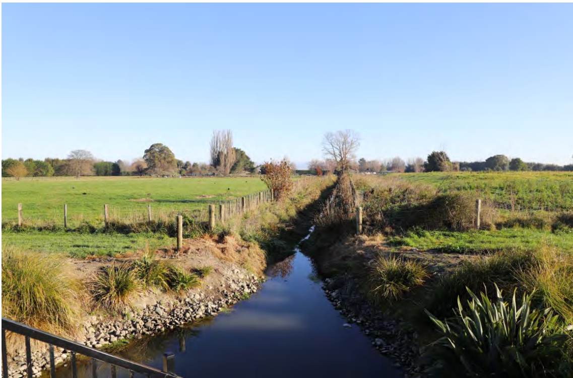
Image 3: Recent upgrades to the stormwater management area in Paddock D.
