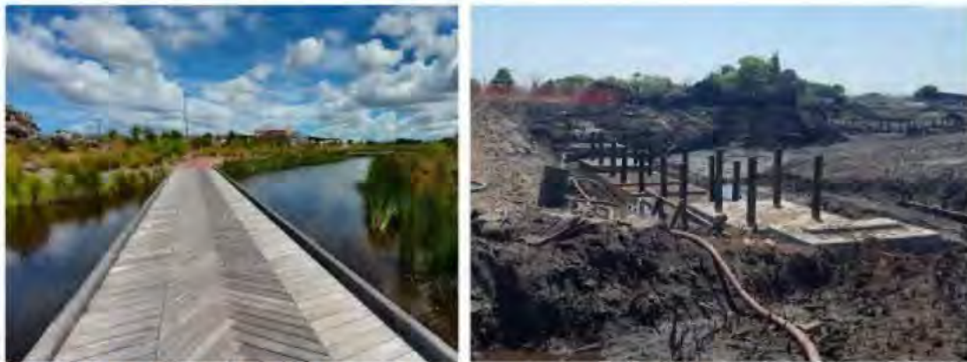
Figure 12 Boardwalk decking (left) and Boardwalk foundations (right)
