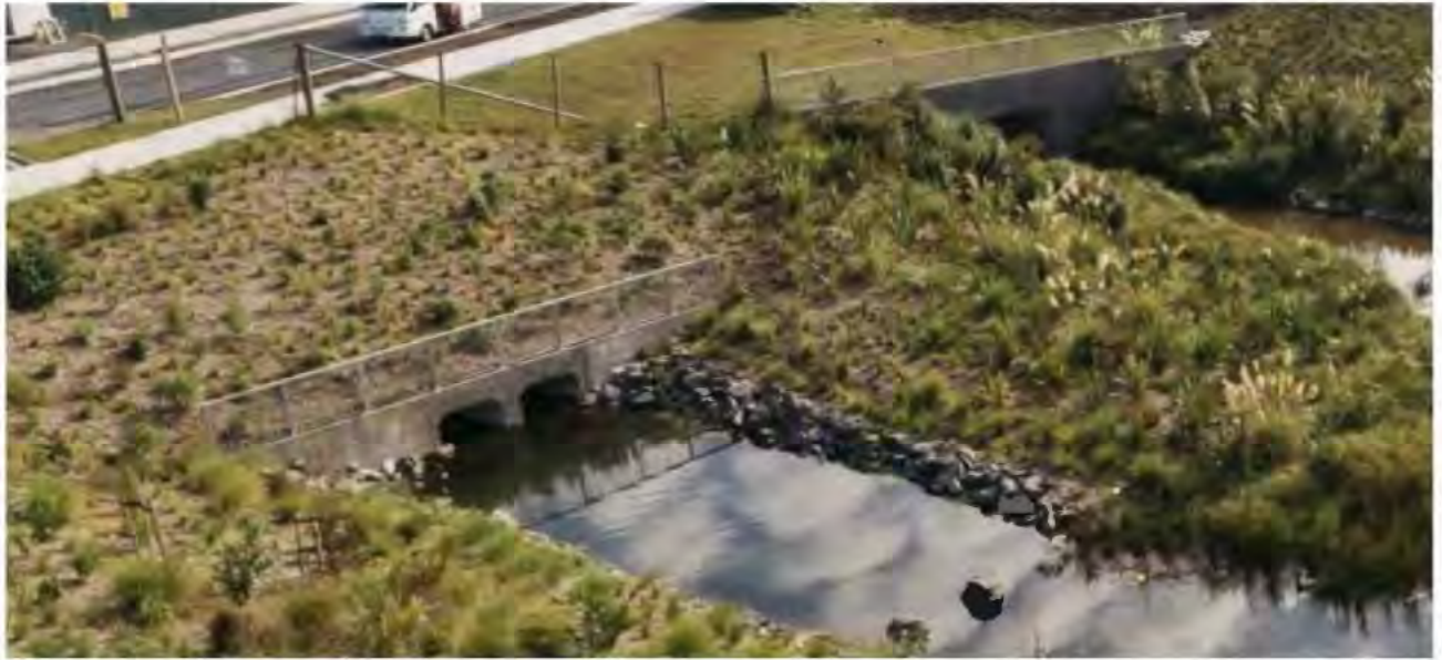
Figure 19 Culvert headwall/wingwalls
