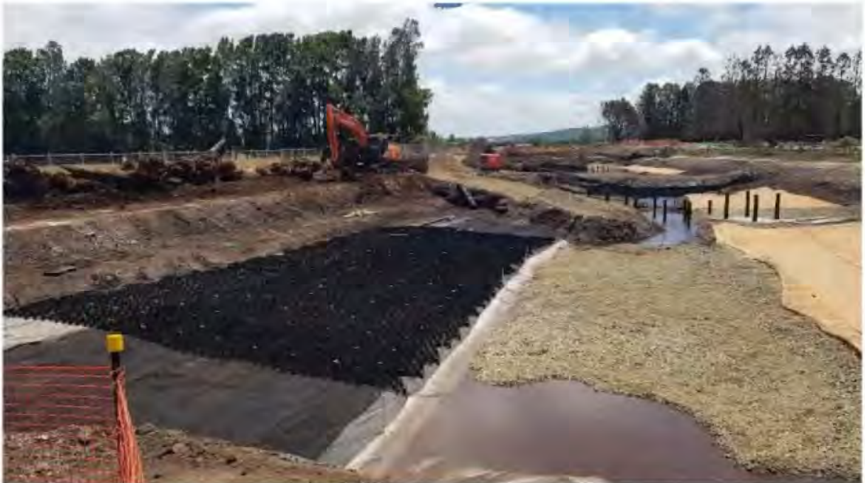
Figure 4 Geoweb scour protection, enkamat and gravel lining for underwater wetland base
