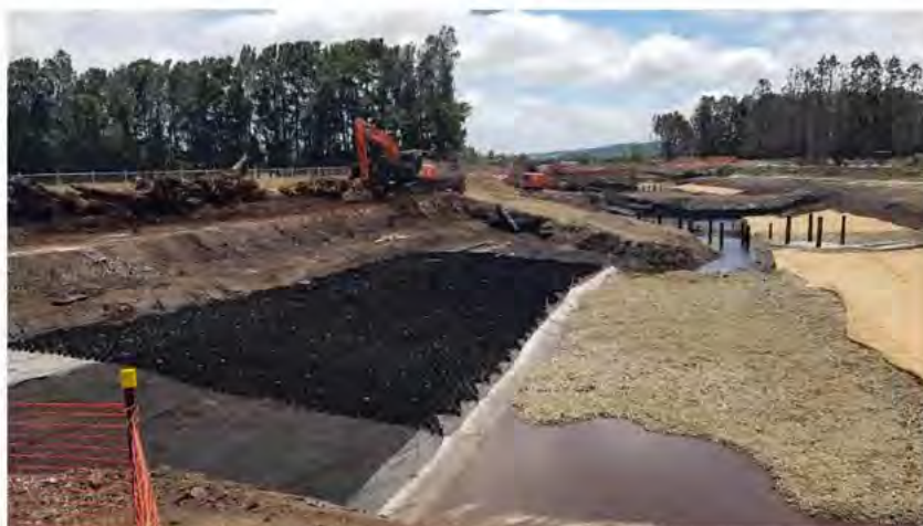
Figure 4 Geoweb scour protection, enkamat and gravel lining for underwater wetland base
