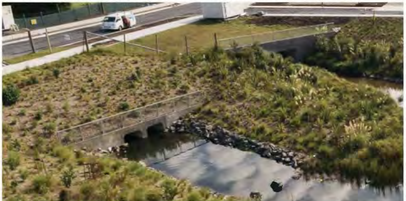
Figure 2 Culvert headwall/wingwalls
