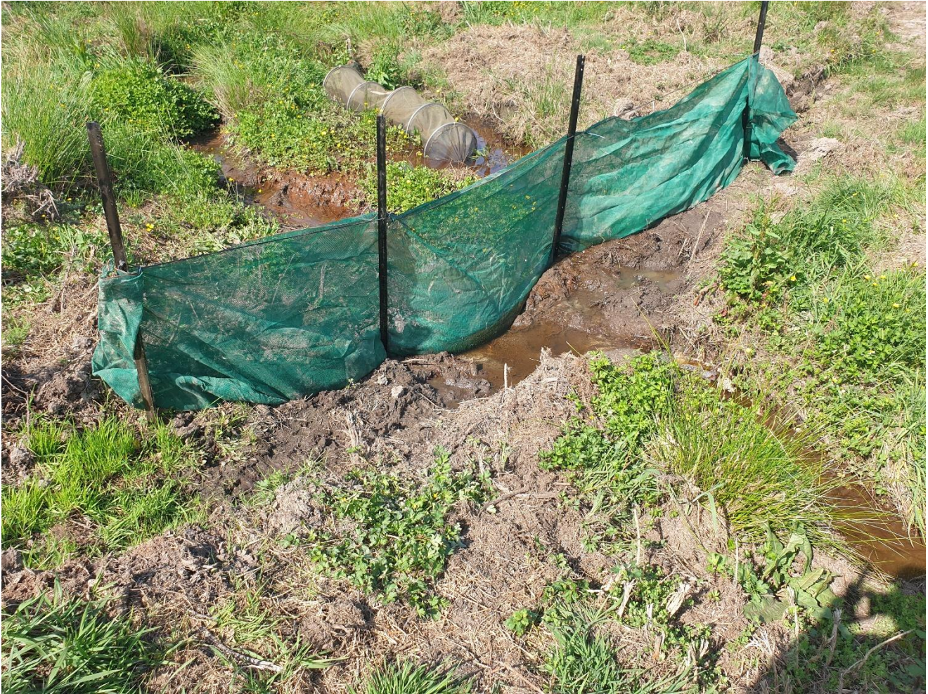
Figure 26. Example photo of fish exclusion screens.
