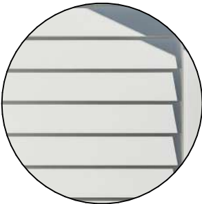
Bevel Back Weather Boards
