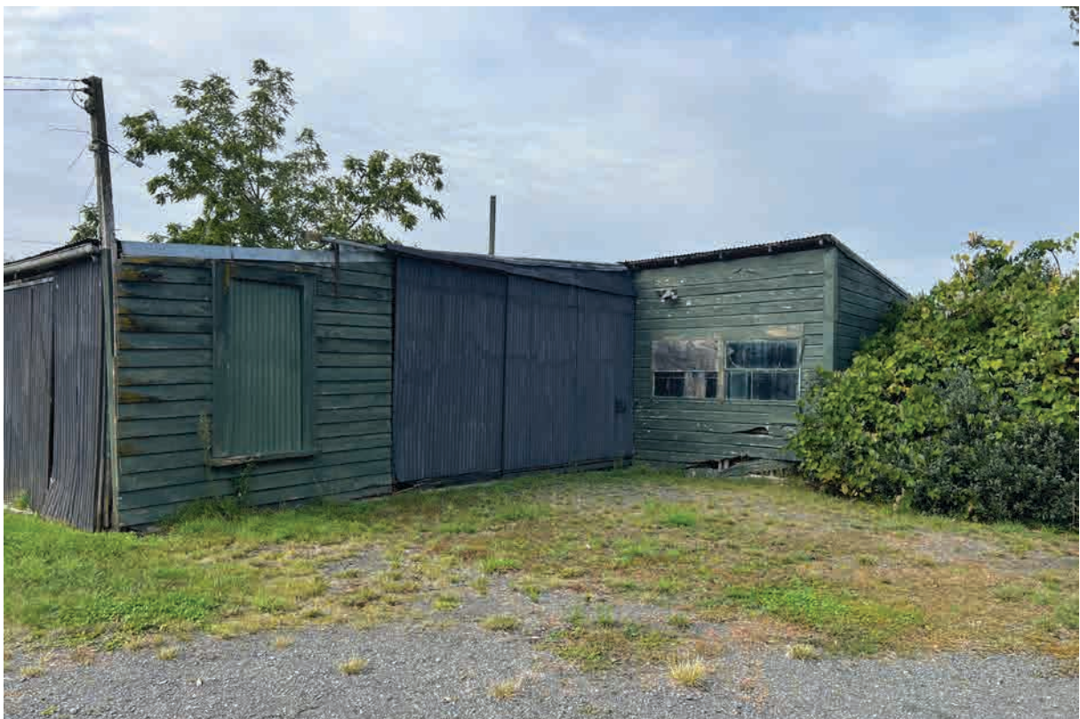
Figure 7. Rear of packing shed, showing lean-to additions.
