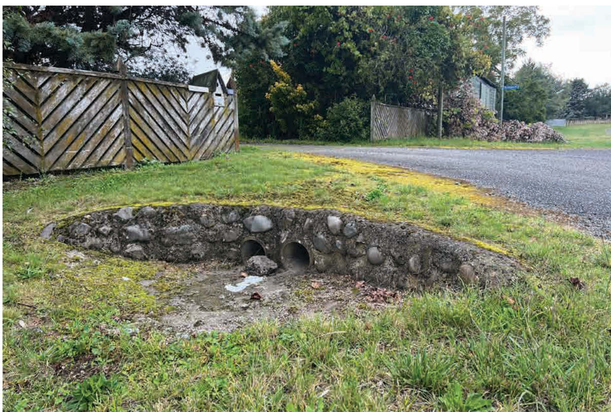
Figure 9. Typical culvert showing header of concrete and river cobbles.
