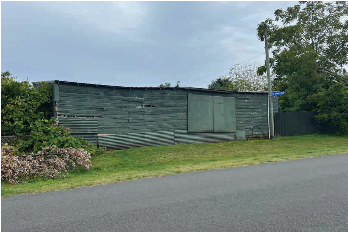
Figure 6. Packing shed from Arataki Road.
