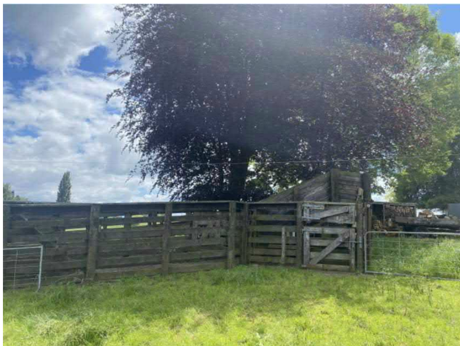
Figure 6.4: Photo of the stockyard at the site.
