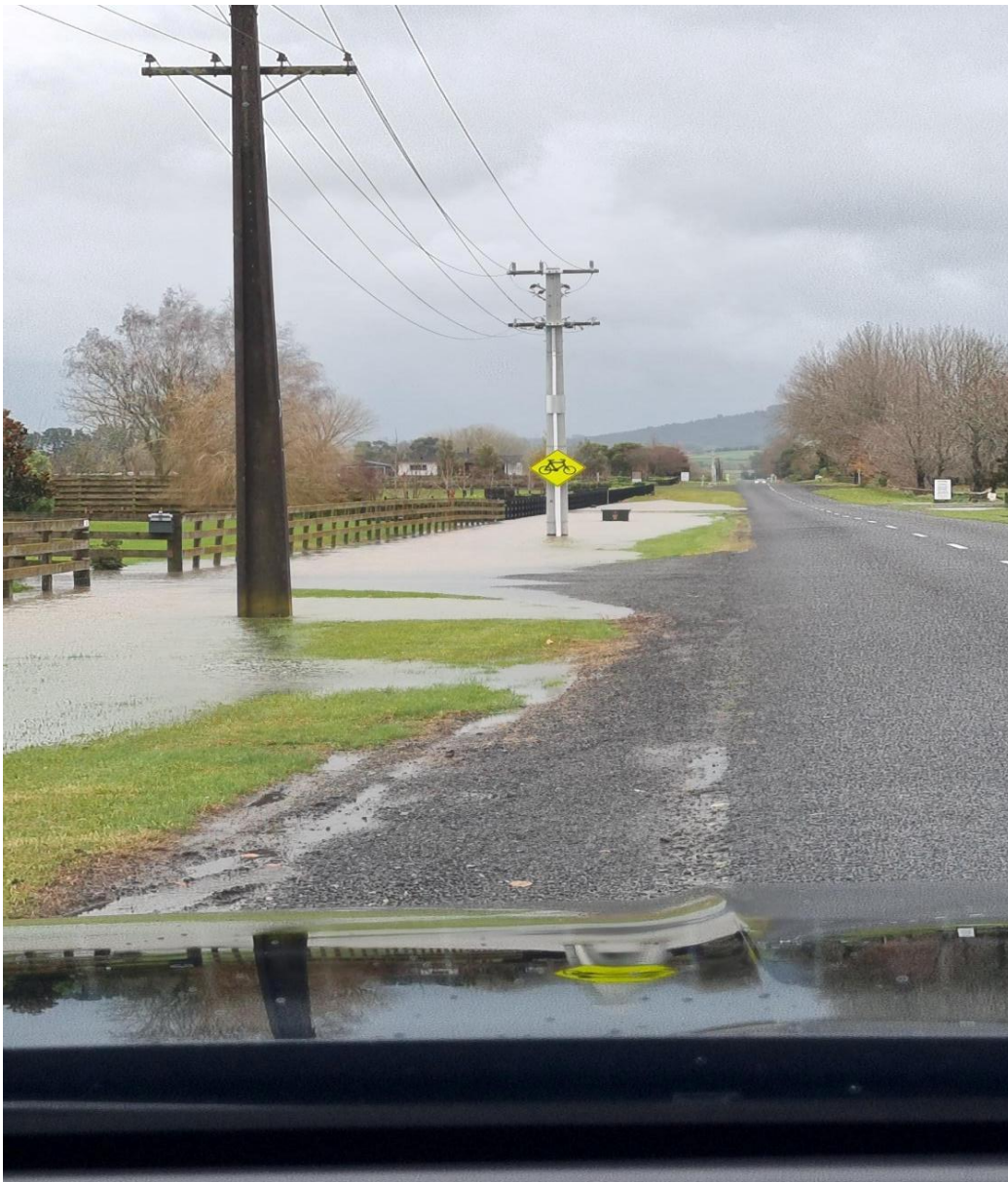
Highgrove Eastern Boundary drain Station road following overnight rain event.
