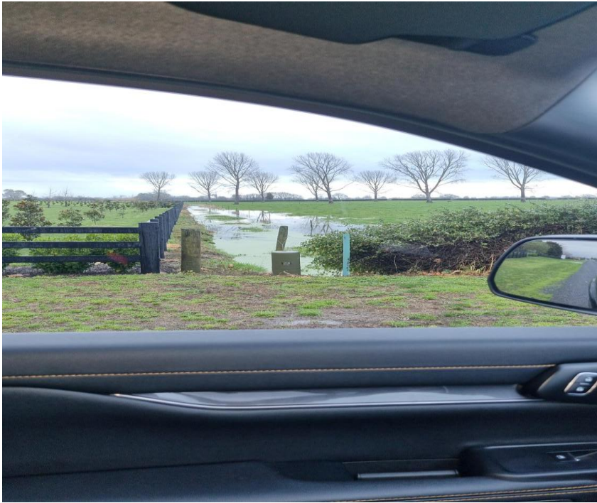
Western boundary of Highgrove/ Ashbourne: Drain overflowing following 50-60mm of rain. This is the location of where the retirement village housing is being proposed to be built at drain level.
