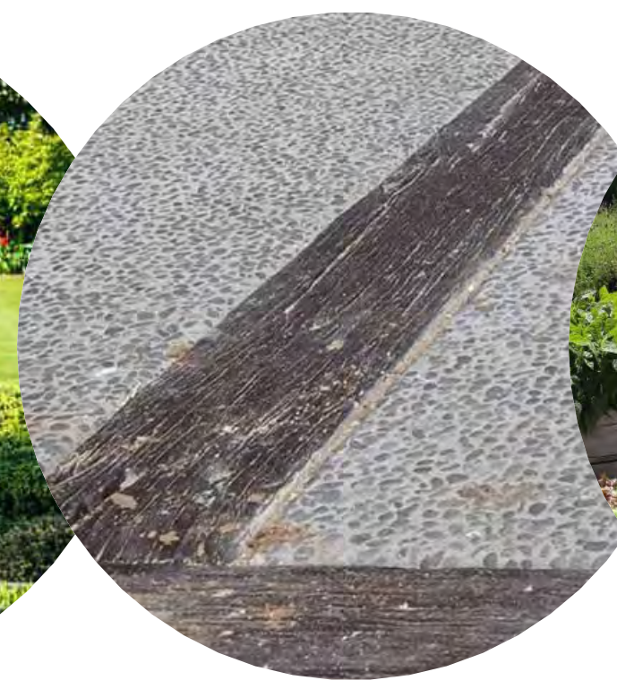
Timber Sleeper in Concrete
