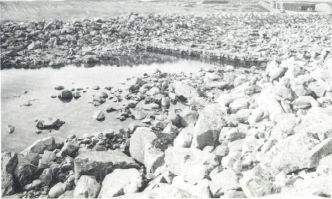
Figure 7: Scour hole downstream of sill 9 which developed after 12 days of tailrace weir and rock chute operation in mid-August 1977
