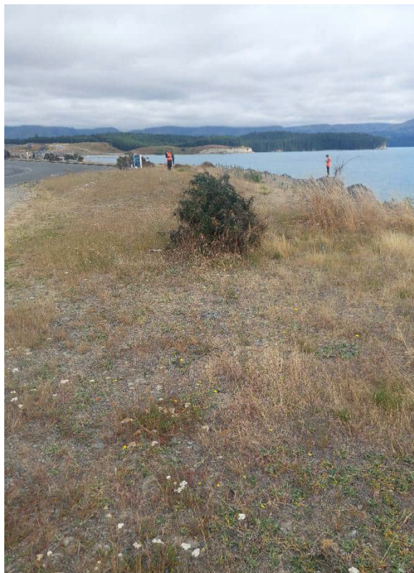
Photograph 2.2: Sparsely distributed vegetation located adjacent to existing dam wall.
