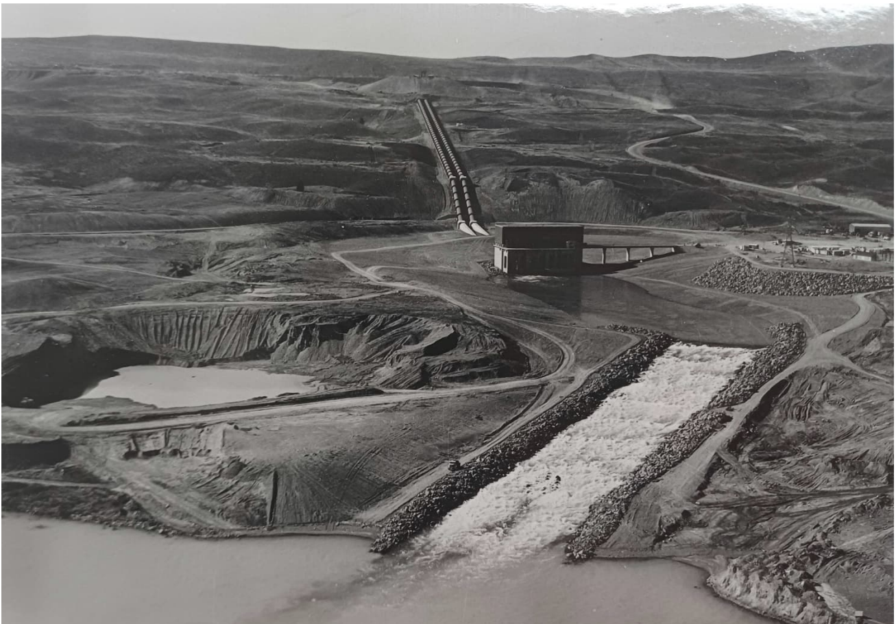
Figure 1-1 Tekapo B powerhouse 1977 (source: Genesis Energy Ltd)
