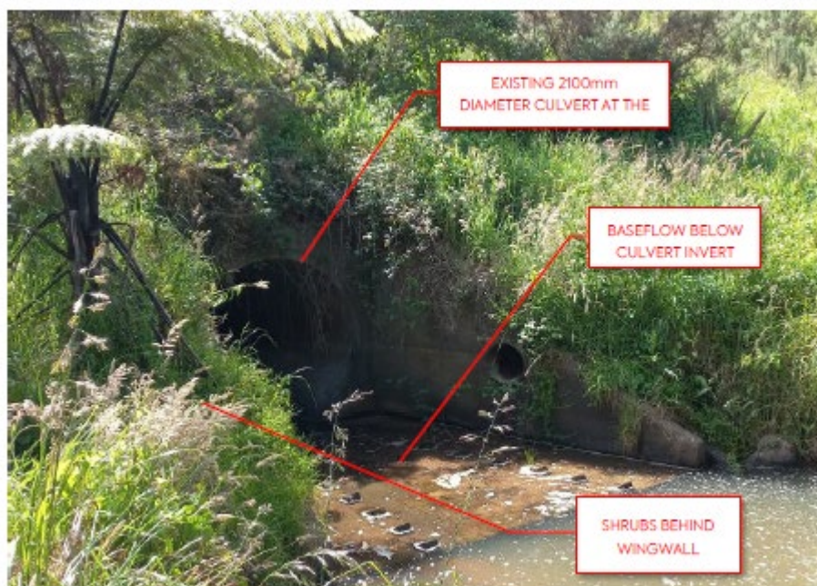
Figure 2: State Highway 1 Culvert (Reproduced from MCKENZIE & CO. Flood Assessment Report)
