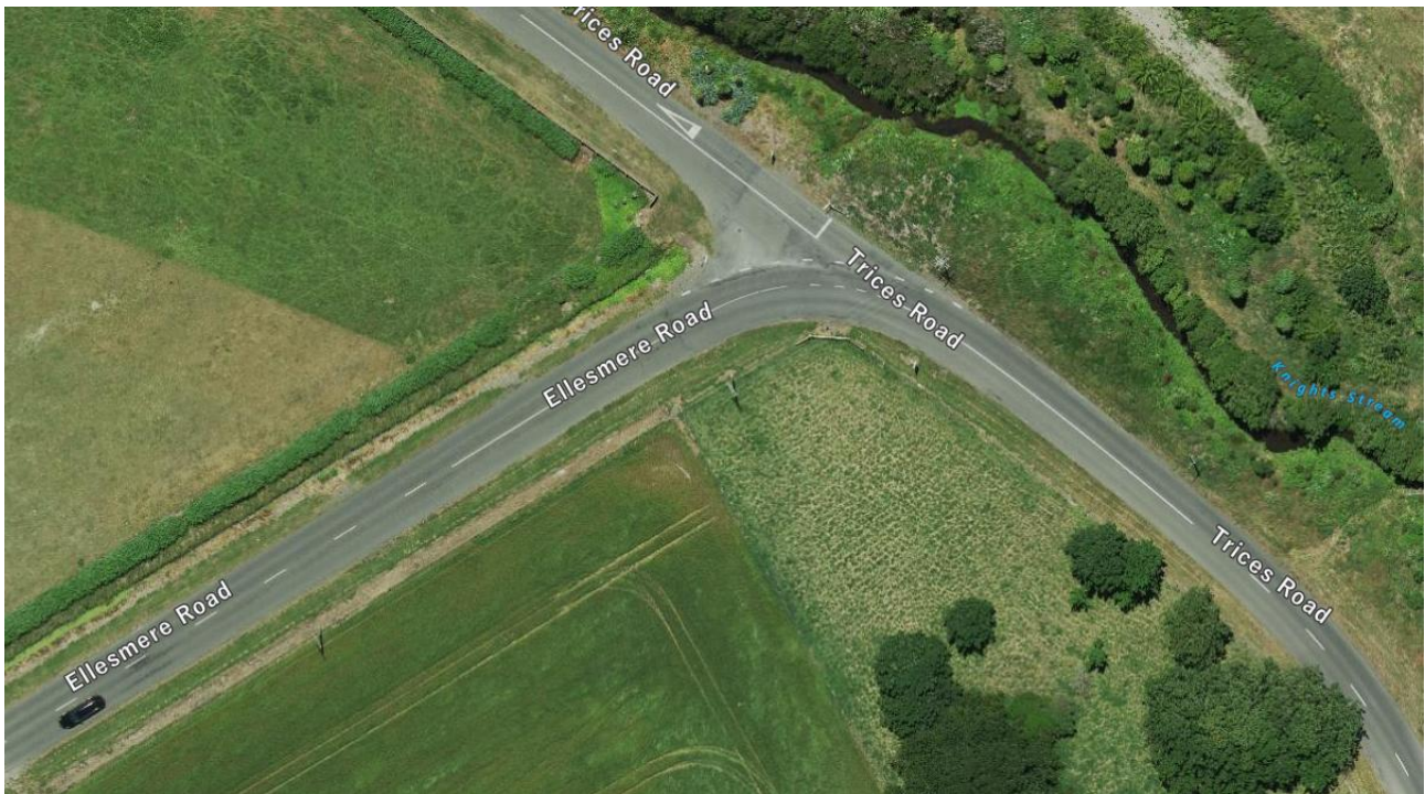
Figure 2.2 Trices Road/Ellesmere Road intersection (Source: Canterbury Maps)
