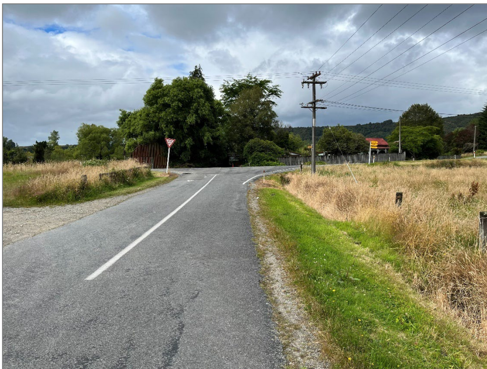
Photograph 4-1: Soldiers Big River Road approach to SH7
