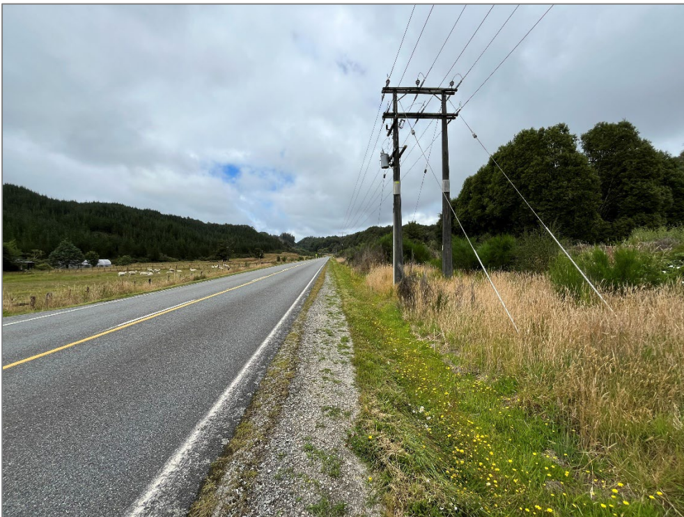
Photograph 7-3: Power poles beside highway near Quigleys Road
