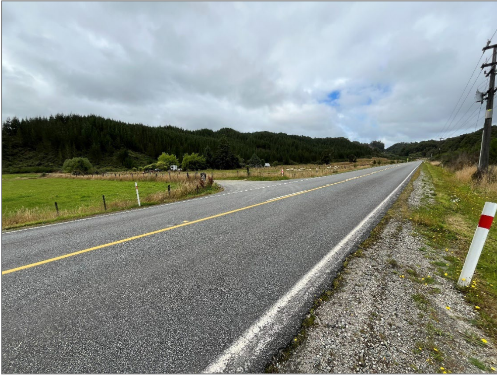
Photograph 4-8: SH7 at Quigleys Road
