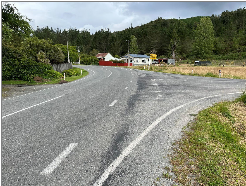
Photograph 3-3: SH7 / Soldiers Big River Road intersection
