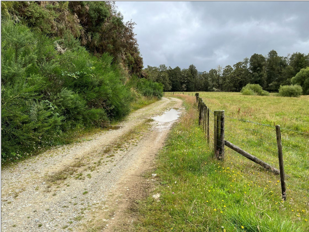
Photograph 4-9: Quigleys Road north of Harwood Road
