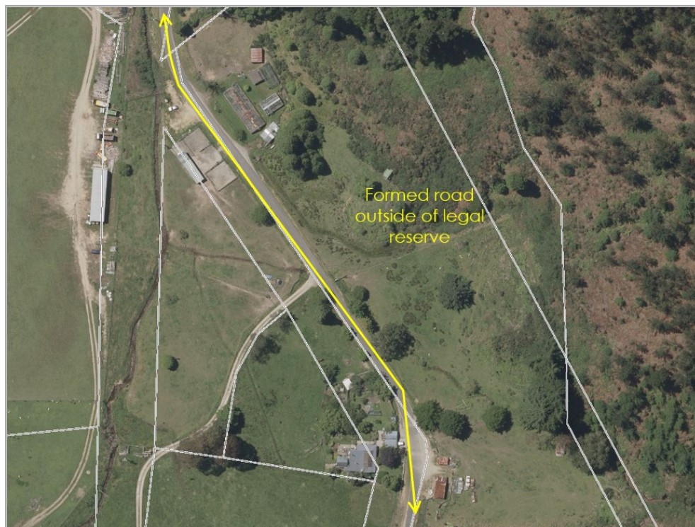
Figure 7-2: Formed road outside legal road reserve
