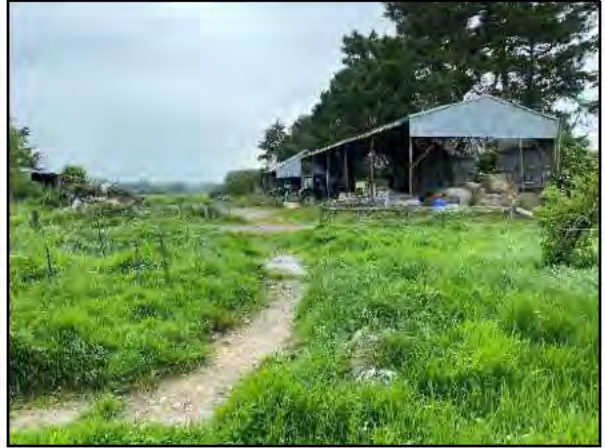
Figure 15: Sheds at S119 from near S120
