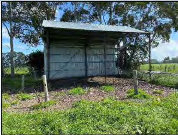
Figure 4: Shed located in the far north-east at S108.
