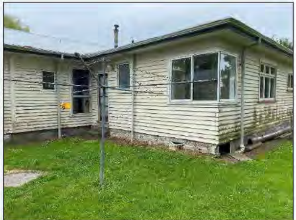
Figure 17: Dwelling near central structures.
