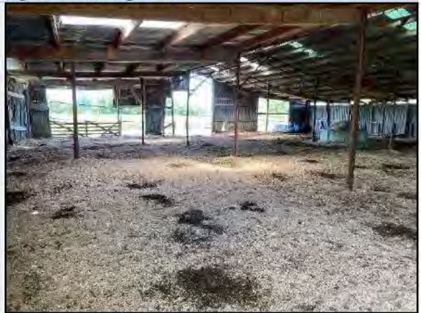
Figure 5: Shed located in centre of site near F-114.
