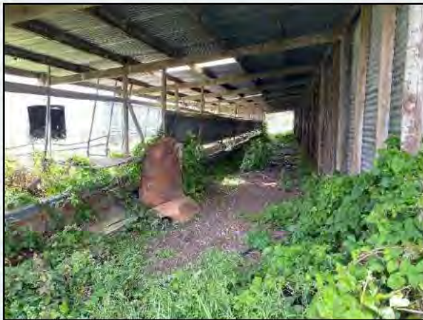
Figure 16: Shed located at S120.
