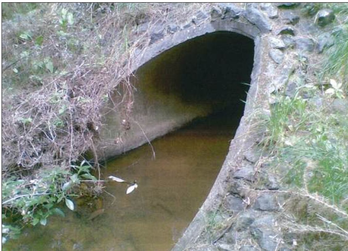
Figure 9: Jack Lachlan Drive culvert.
