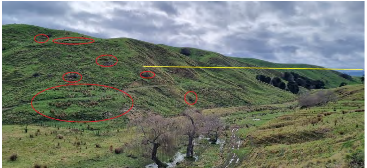
Figure 11: View of northern abutment of proposed dam. Approximate dam centreline shown in yellow and areas of rushes circled red. Pouarua River meander in foreground.
