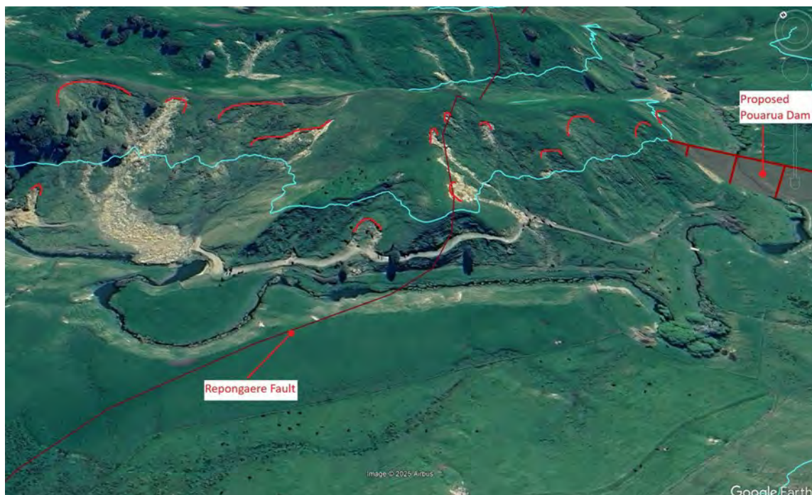
Figure 24: 2025 Google Earth image showing extent of slope instability/landsliding on norther valley slopes. A selection of both historic and recent landslide scarps shown in red.
