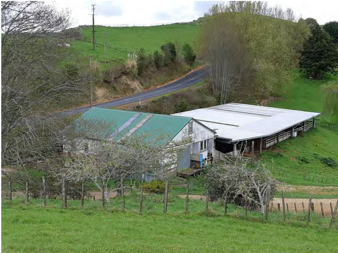
Photograph 10: View of Building 2 facing south on the southern site boundary. Building used as wool shed (for shearing), livestock pen and livestock spraying area; Oparure Road is visible beyond the building.
