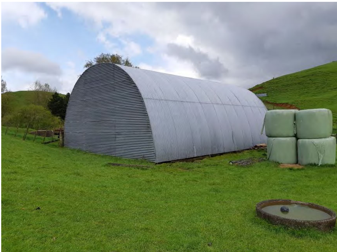
Photograph 8: View of Building 1 facing south west in the southern section of the site. Building used for storing a tractor and farming equipment.
