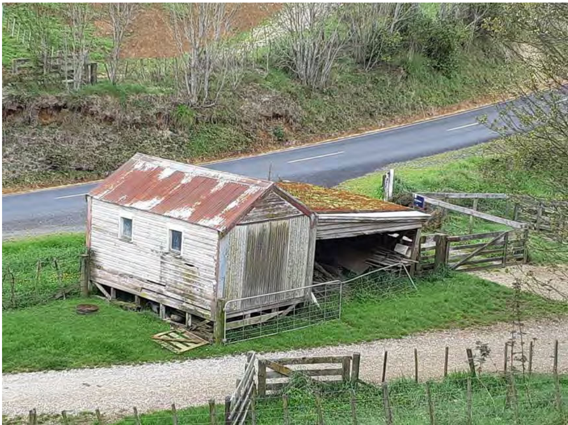
Photograph 14: View of Building 3 facing south on the southern site boundary; Oparure Road is visible beyond the building. Building used to store wool off cuts.
