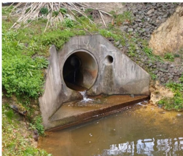
Figure 1 Existing Watercourse 1 outfall from existing 900mm pipe
