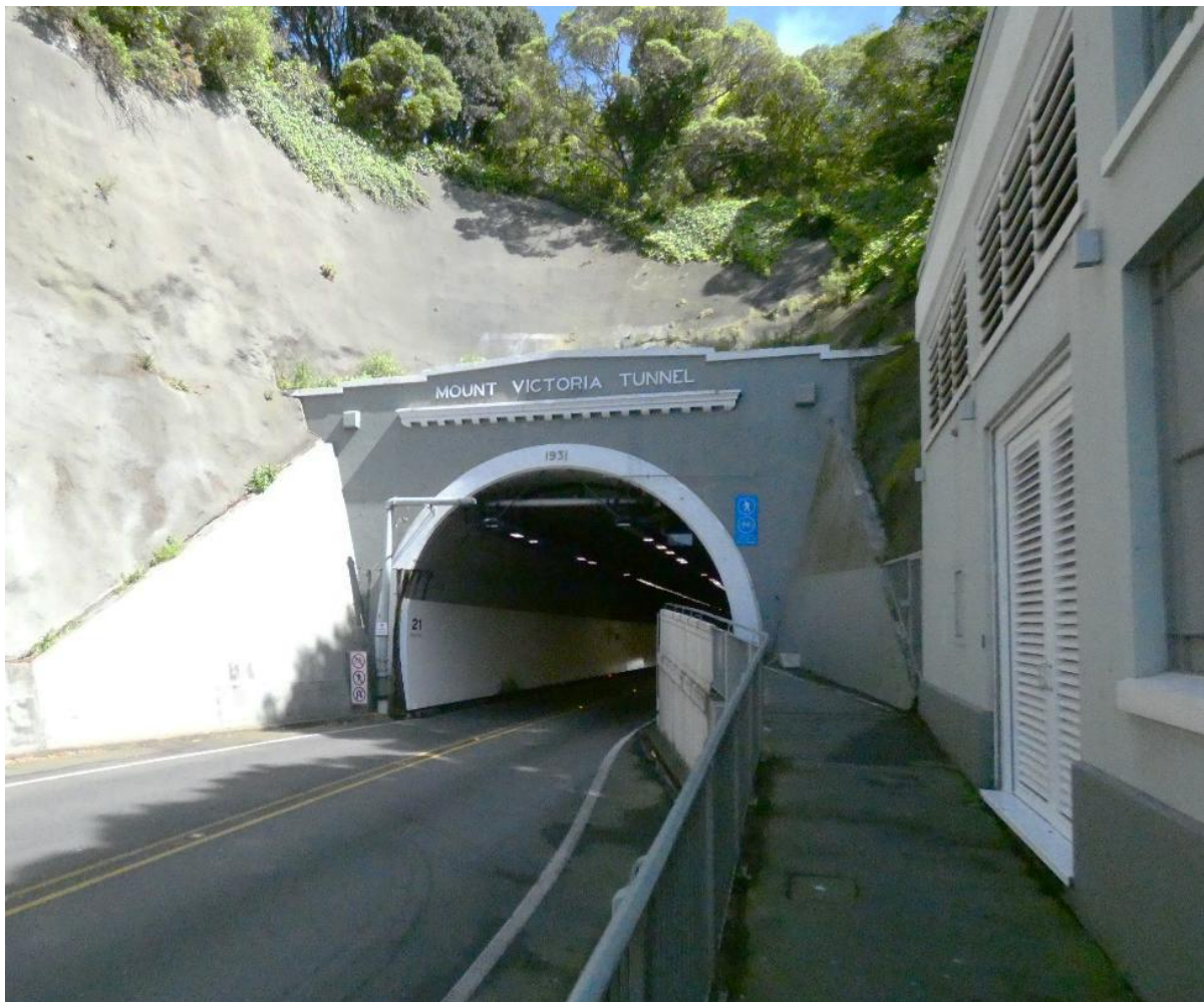
Figure 6 – Existing eastern entrance to Mt Victoria Tunnel
