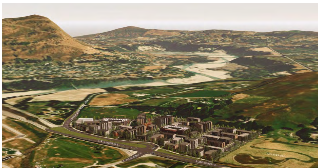
Image 1: Aerial view of the Project, prepared by Brewer Davidson, (SK09 rev 02, 9/07/2026).
