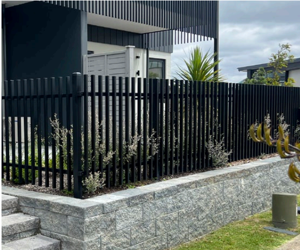
1-1.2M HEIGHT SLATTED FENCE USE: JOAL AND STREET FACING BOUNDARIES WHERE LESS PRIVACY REQUIRED
