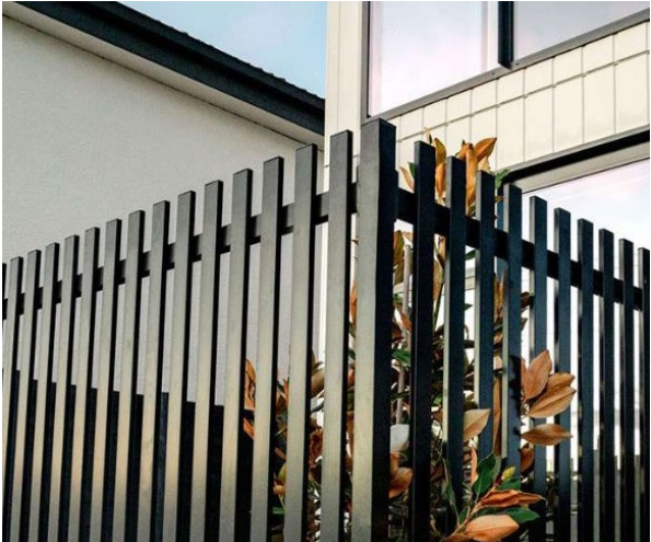
1-1.2M HEIGHT SLATTED FENCE USE: JOAL AND STREET FACING BOUNDARIES WHERE LESS PRIVACY REQUIRED
