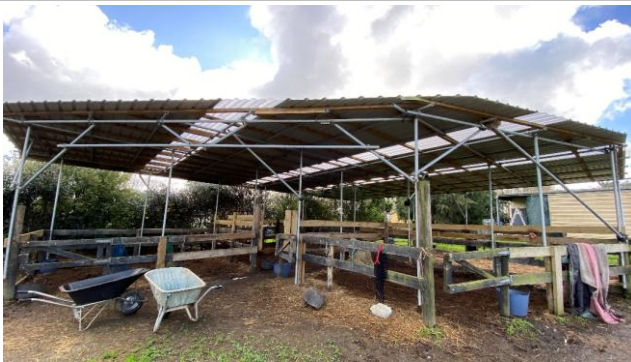
Photograph 13. View of the covered yards, facing northeast.
