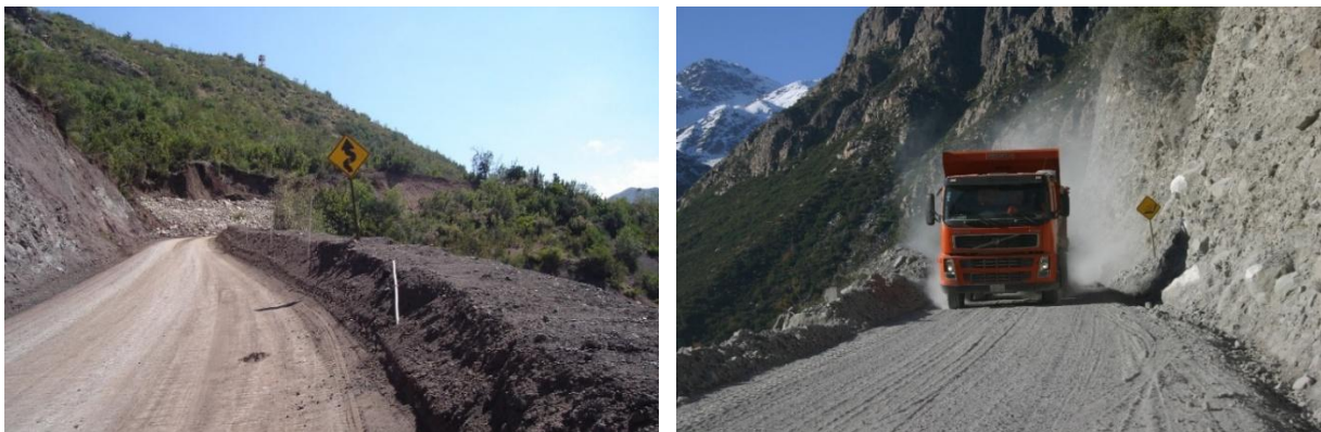
Figure 19: Examples of edge protection, Chile, elevation 2850 m
