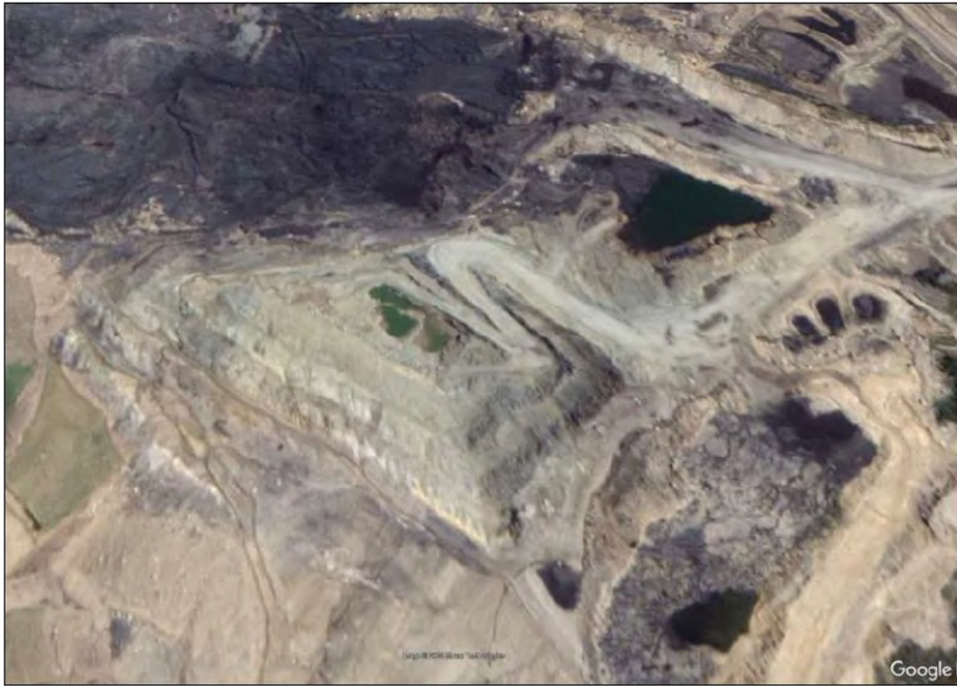
Figure C4: Google Earth 7/1/2018 – Water beginning to accumulate in base of A-Drive borrow pit.
