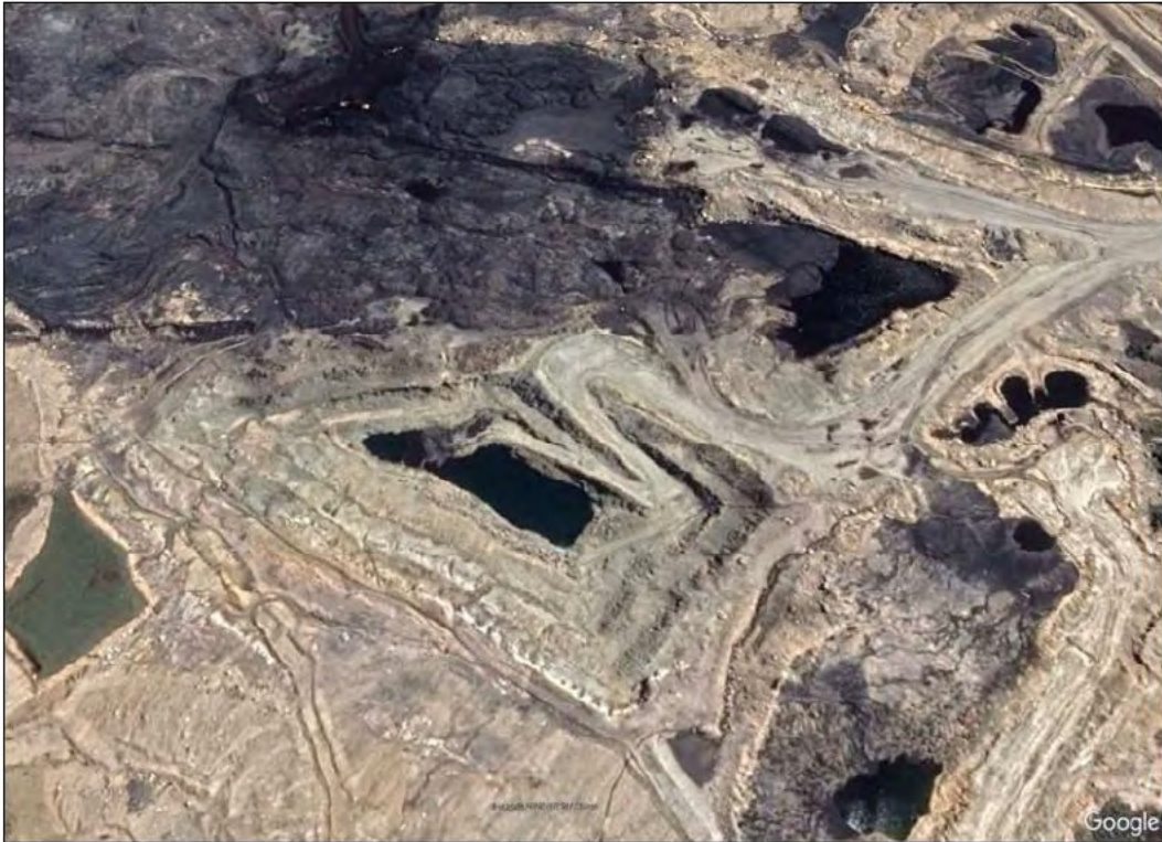
Figure C6: Google Earth - 8/1/2019 – A-Drive borrow pit filling with water.
