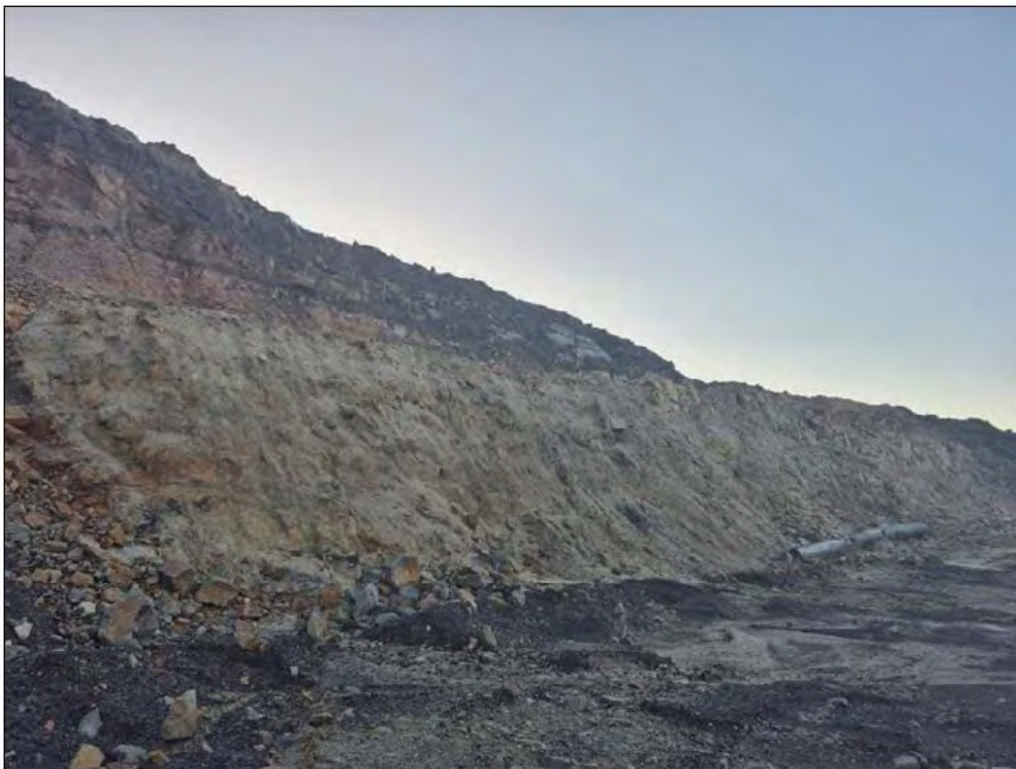
Figure B6: Photograph of the northern highwall of the A-Drive borrow pit. Note: Surficial layer (approximately 1.0 m thick) of completely weathered to extremely weathered granite on highwall batter face.
