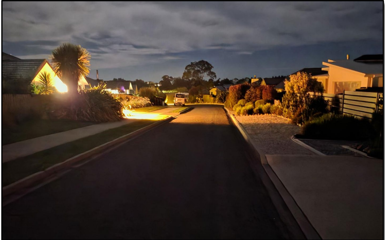
Figure 11: Bollard Lighting (35 metres) Koi Crescent in Tasman.
