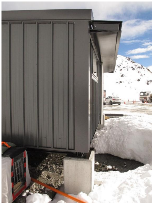
Figure 14. Patrol Building on Elevated footings above potential flood level
