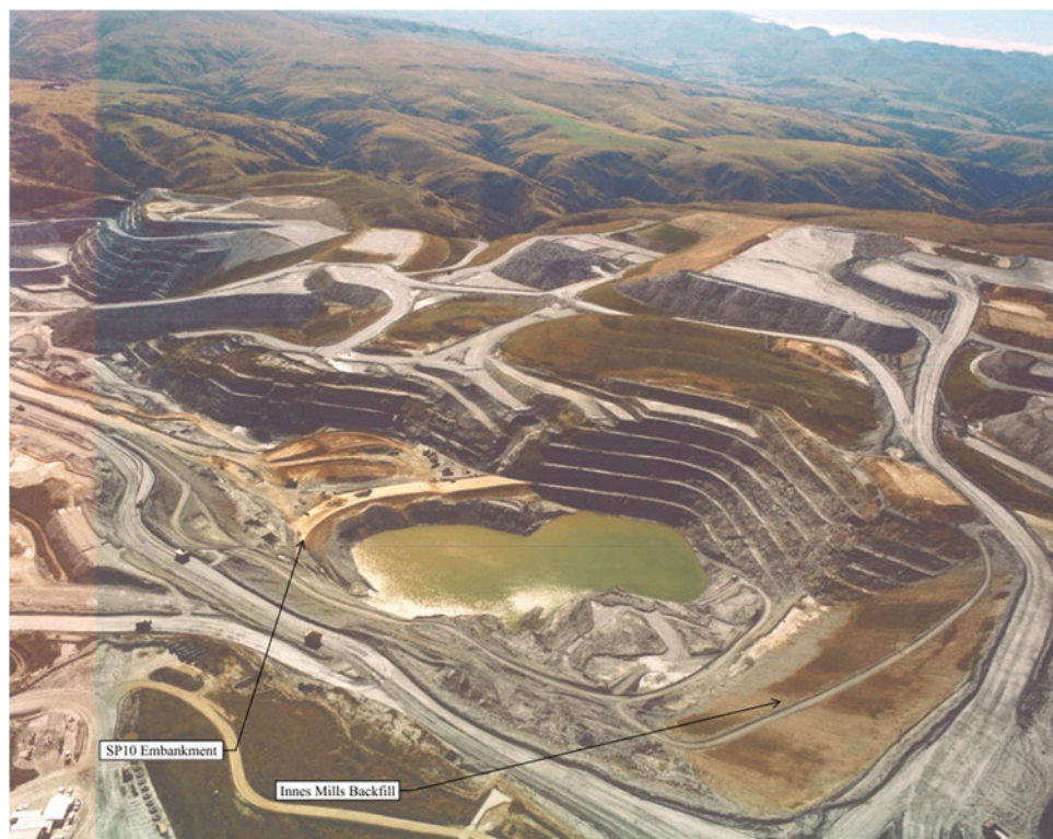
Figure 5: Aerial photo showing SP10 Zone A being placed at the upstream toe of the SP10 embankment in 2002
