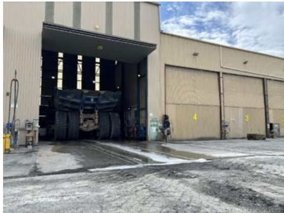
Photograph 1. Eastern side of Main Workshop, wash water draining to slot drain
