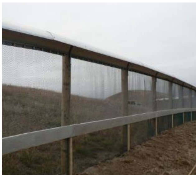
Figure 8: A full height pest exclusion fence (as constructed by Pestproof Fences Ltd).
