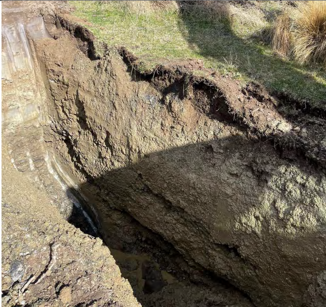
Testpit at completion. Max depth 4.4m
