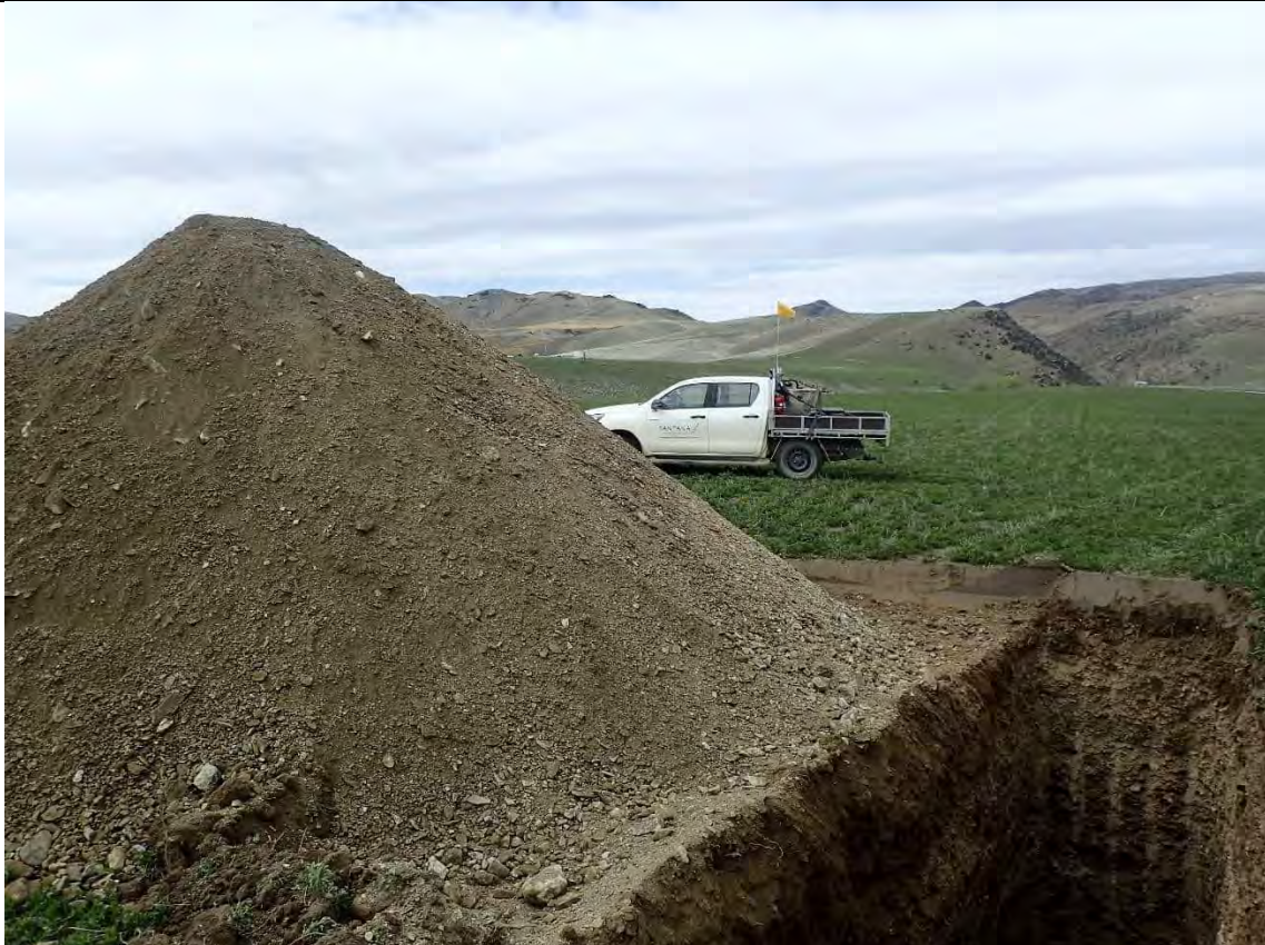
Testpit at completion. Max depth 7m
