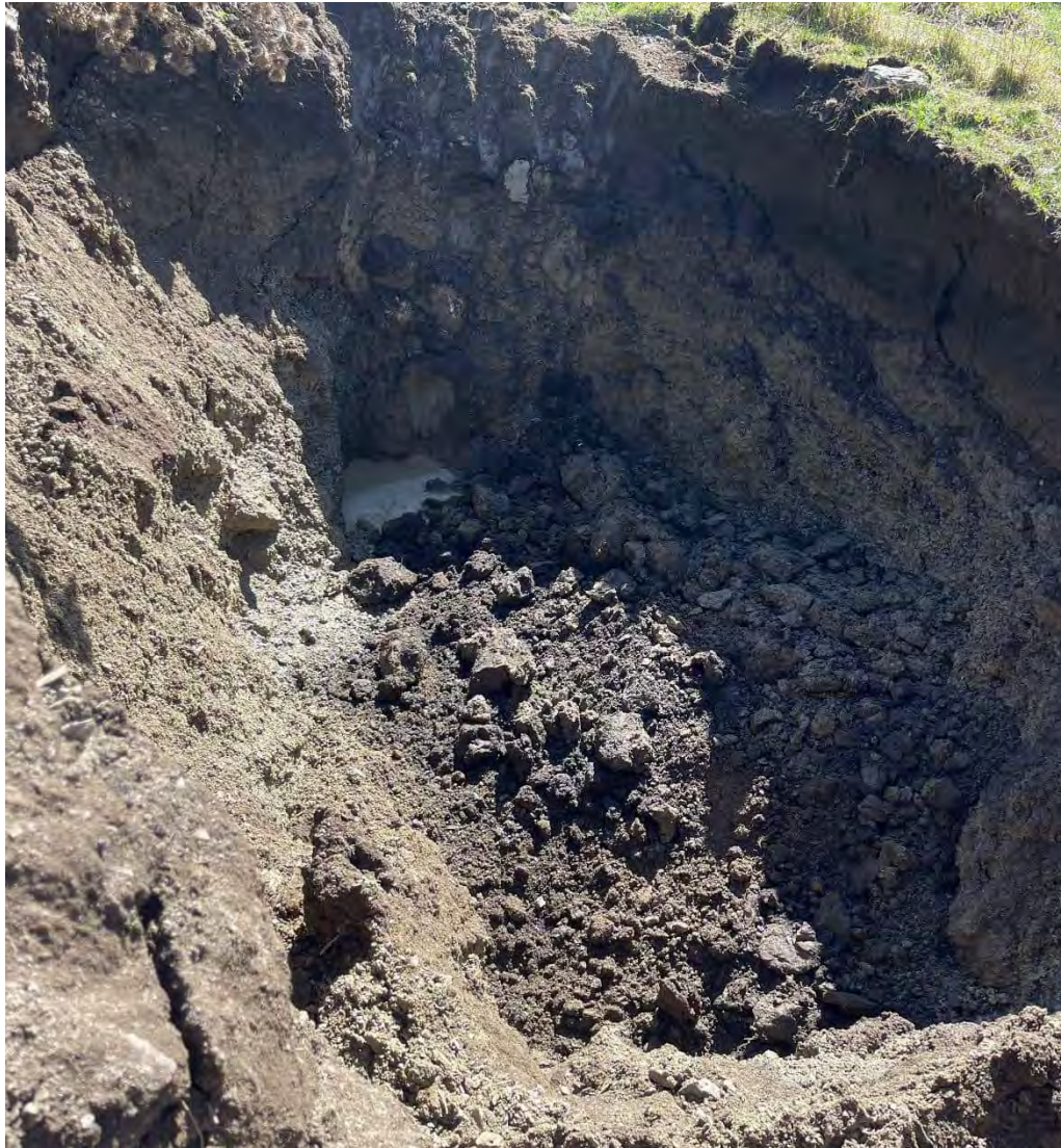
Testpit at completion. Max depth 3m
