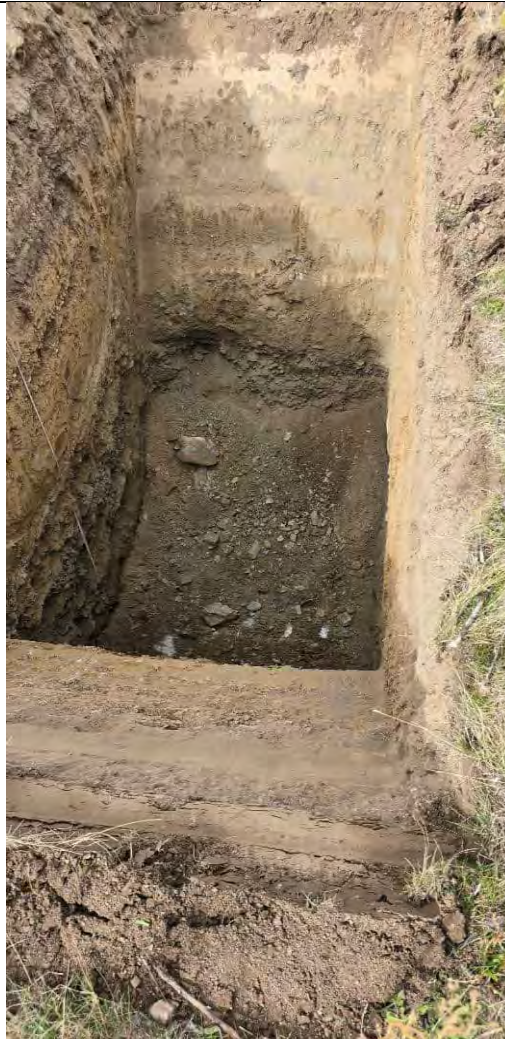
Testpit at completion. Max depth 3.6m
