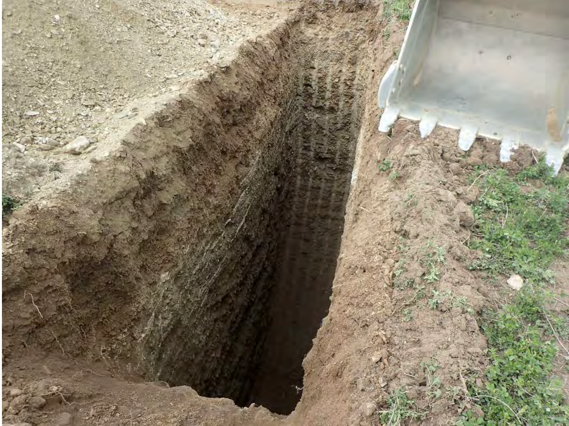
Testpit at completion. Max depth 6m
