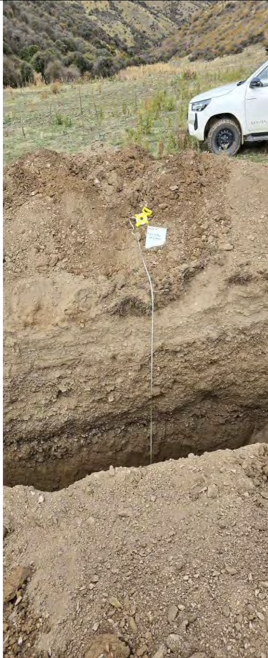
Testpit at completion. Max depth 3.2m
