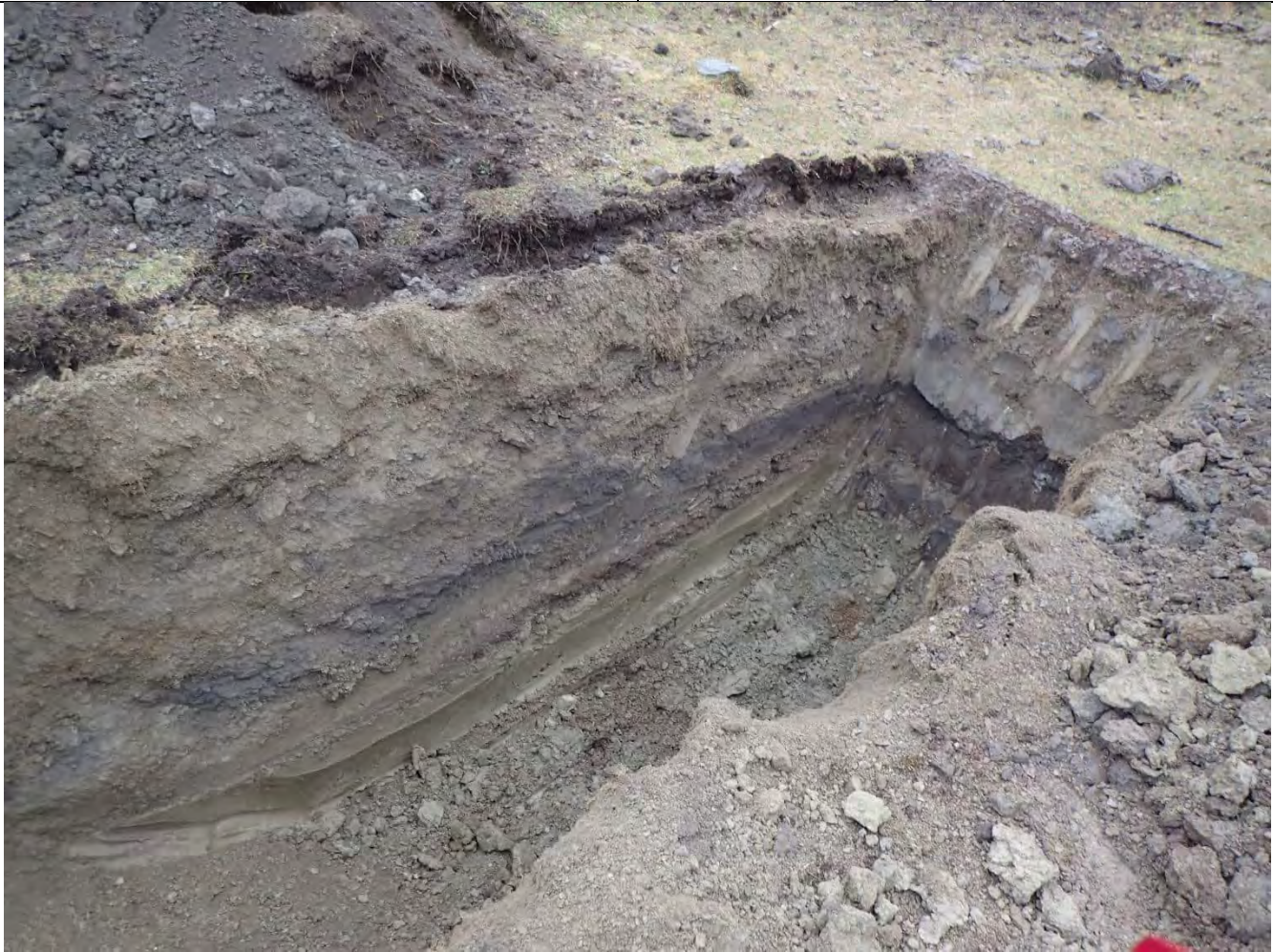
Testpit at completion. Max depth 1m
