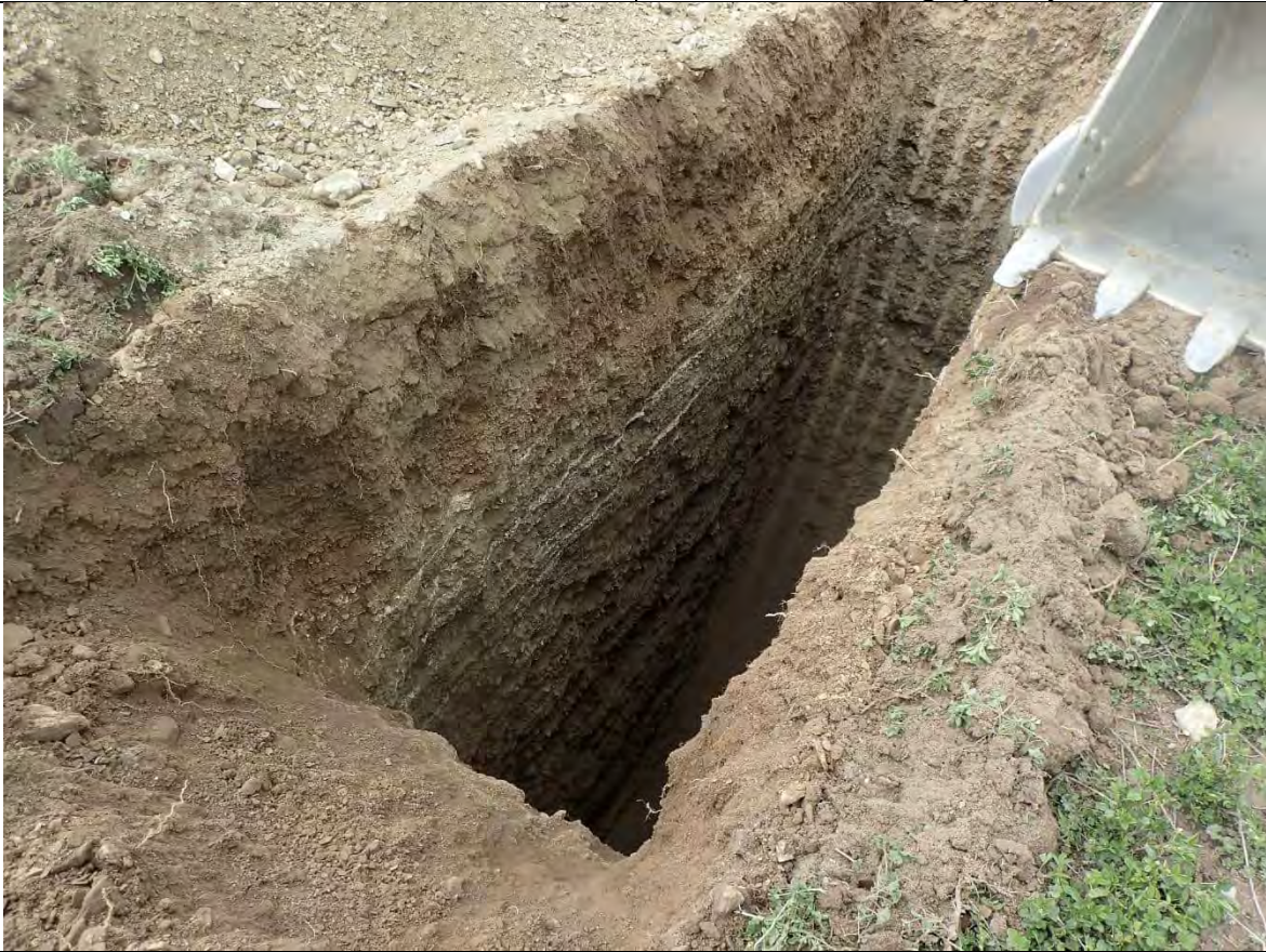
Testpit at completion. Max depth 7m
