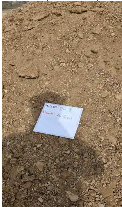
Spoil pile at end of excavation.
