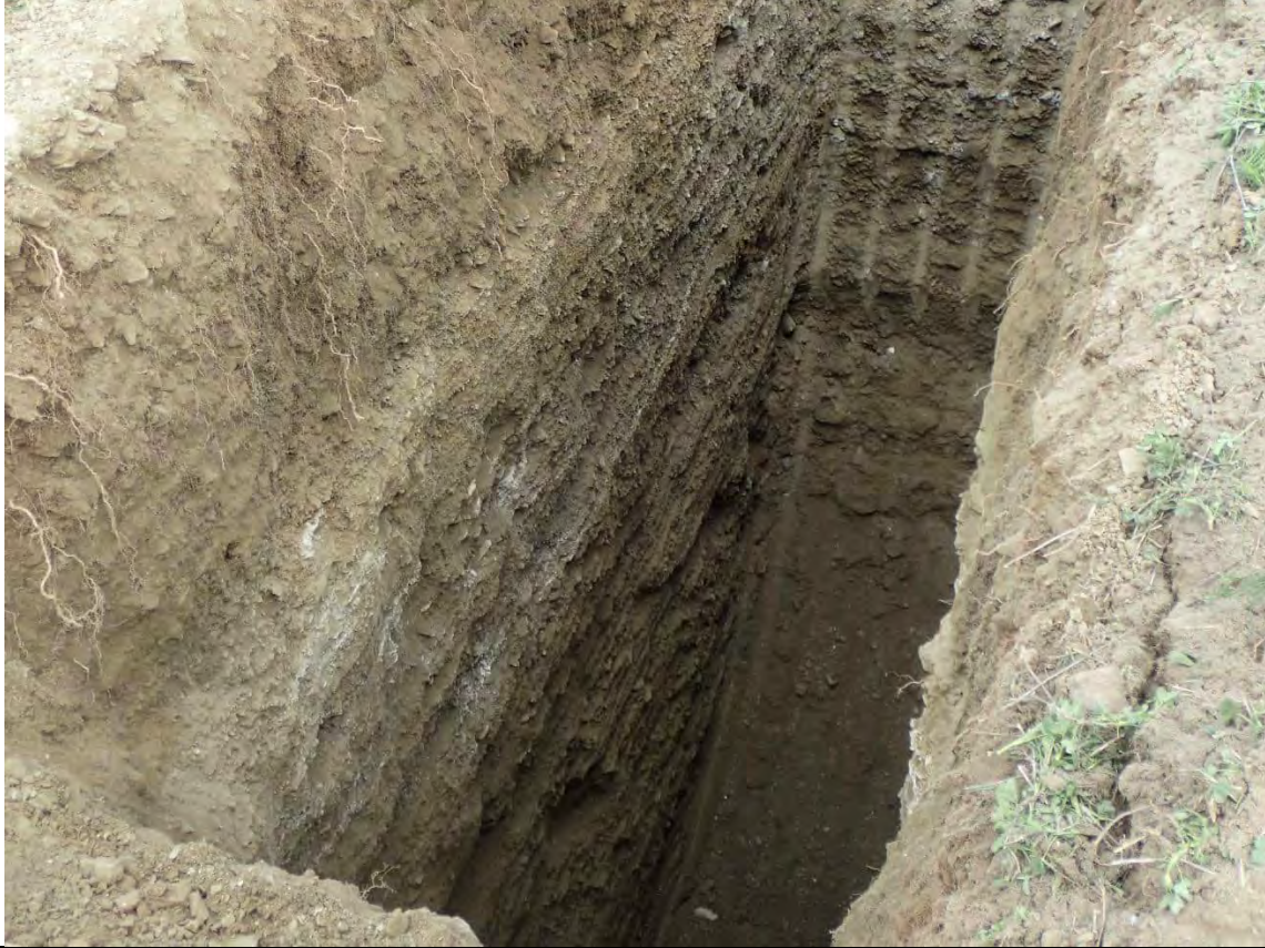
Testpit at completion. Max depth 6m
