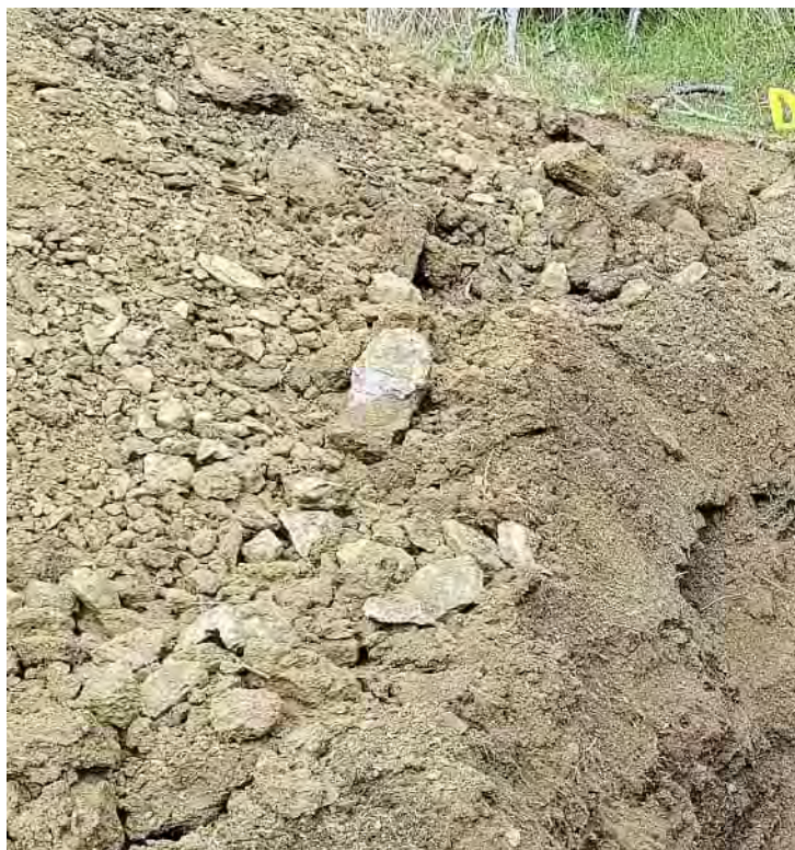
Spoil pile at end of excavation
