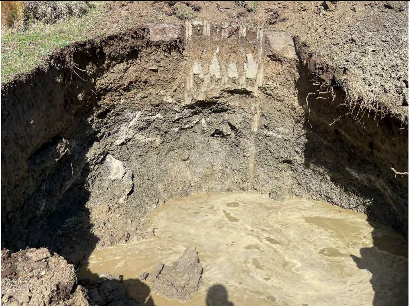
Testpit at completion. Max depth 5m
