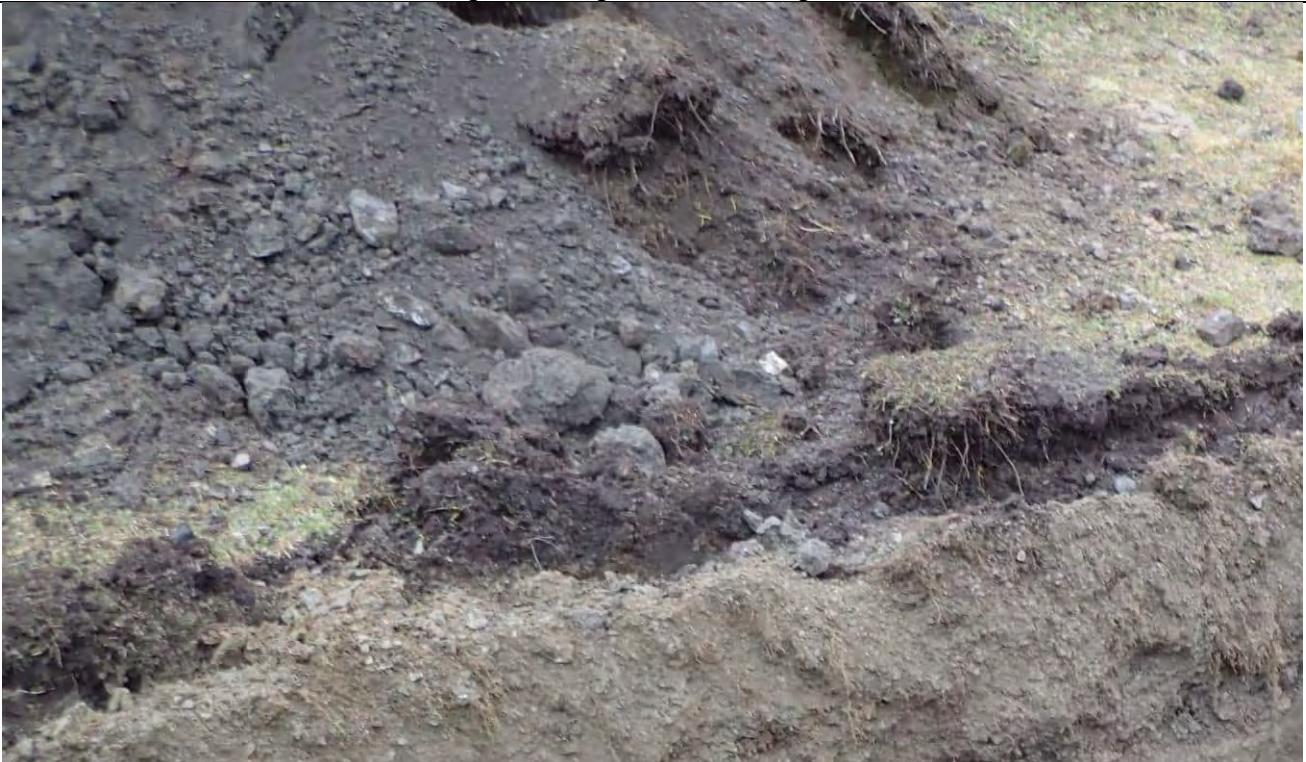
Spoil pile at end of excavation
