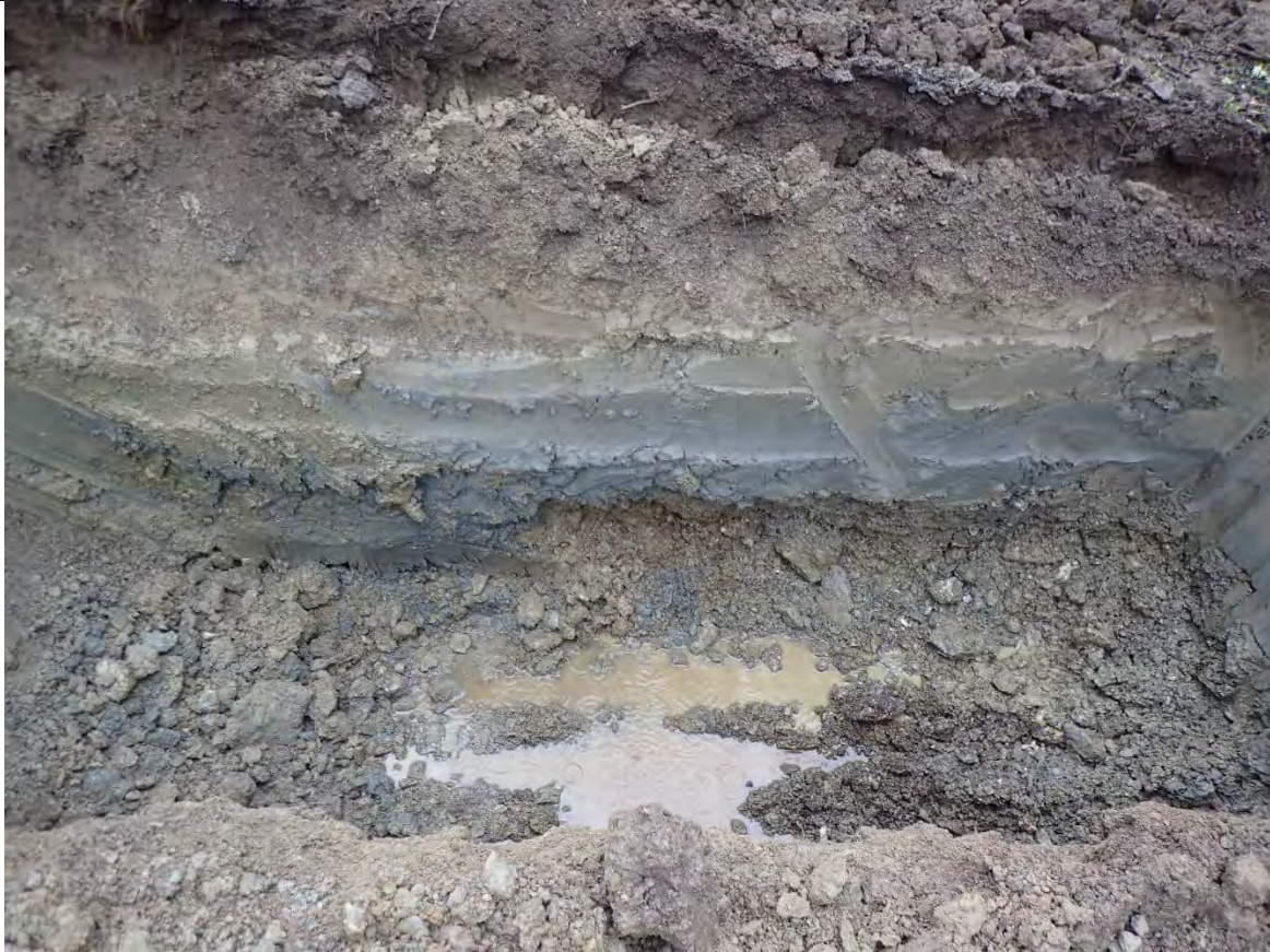
Testpit at completion. Max depth 2.5m
