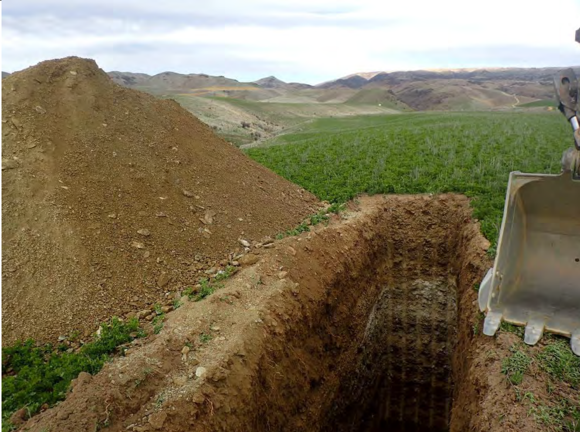
Spoil pile at end of excavation
