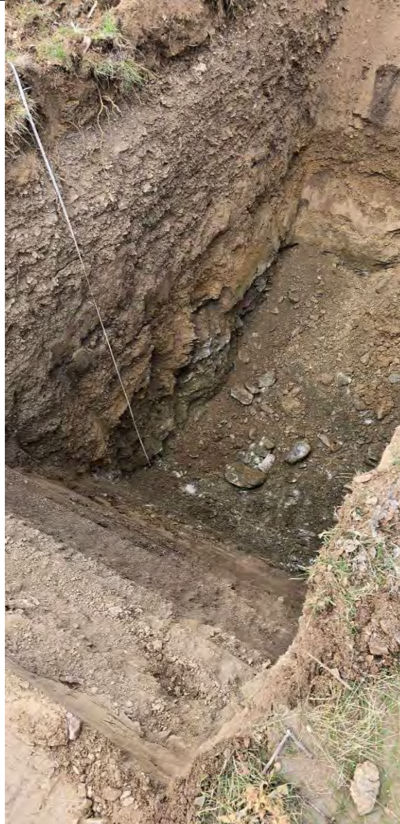
Testpit at completion. Max depth 3.8m
