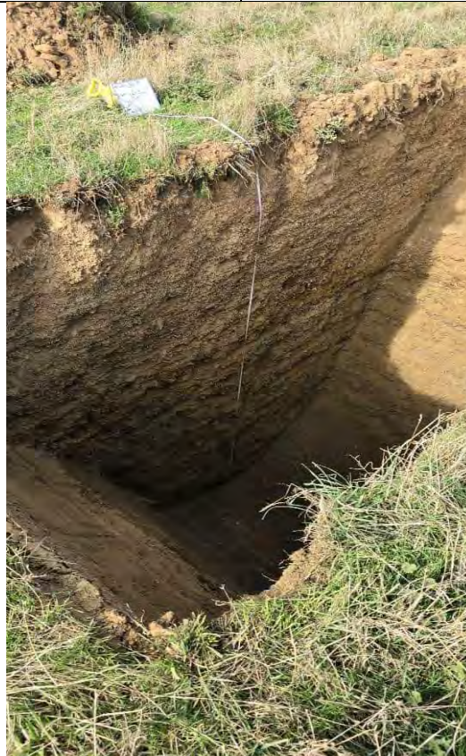
Testpit at completion. Max depth 4.2m
