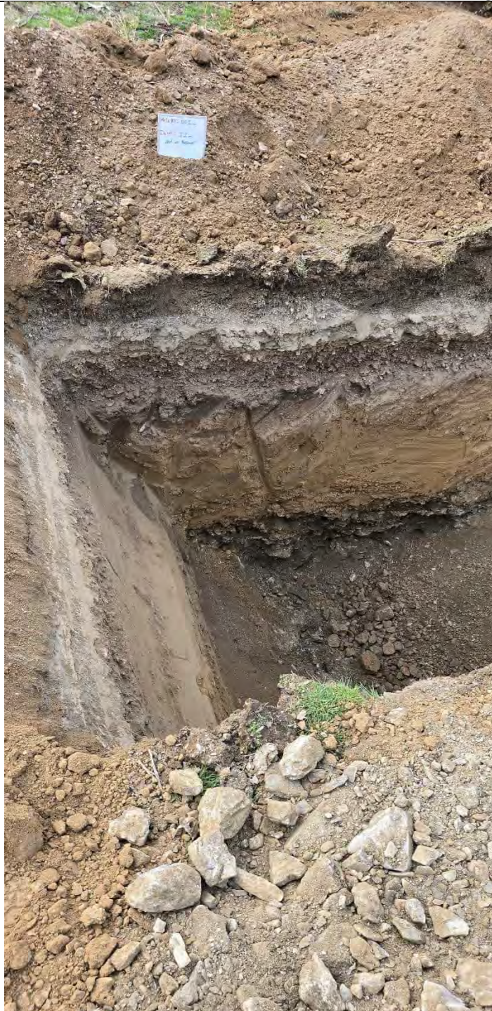
Testpit at completion. Max depth 3.1m
