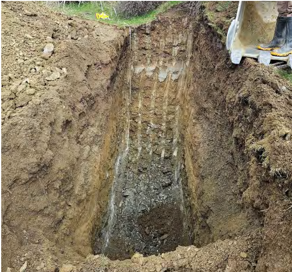
Testpit at completion. Max depth 5m
