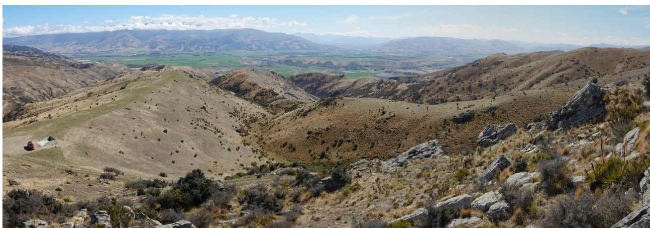
3.. Panorama view of diversion ridge from above airstrip
