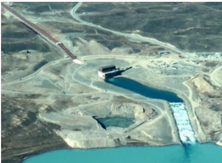
Figure 2 - Exposed Tekapo temporary tailrace and weir following construction
