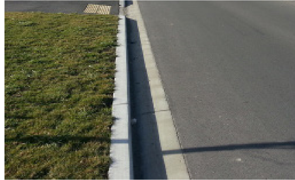
Insitu concrete kerb & channel
