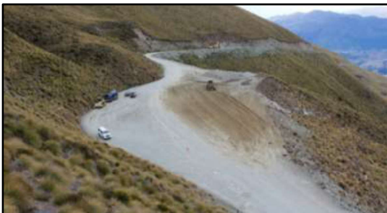
Figure 78. Note the rehabilitation below the road and beside the parked vehicles. Also the far corner has been cut and replanted.
