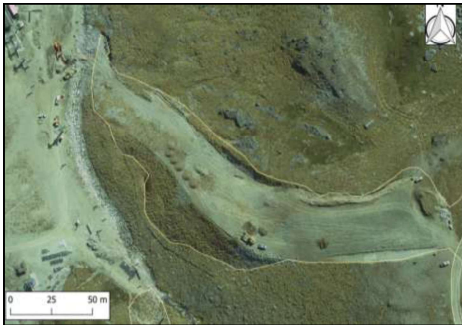
Figure 74. Aerial view of the recent work (refer Figure 71 above) withreworked area outlined in yellow and replanted area the slope below he skin trail. Note piles of saved top soil and repainted tussocks on the trail.
