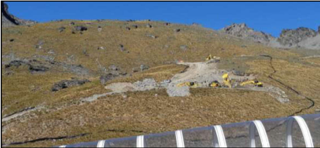
Figure 71. Sugar Bowl trail 2020 under construction. The area enclosed by the black fence and the track above has been reshaped and revegetated by machines and is hardly distinguishable from the untouched tussock grassland.
