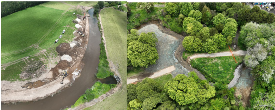
Waiari berm and channel desilting
