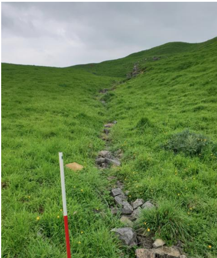
Figure 27. Rock-filled farm drains
