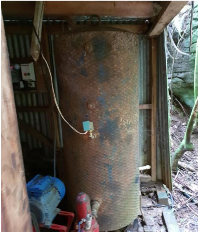
Figure 26. Pumphouse in the entrance of the Guildford Cave system
