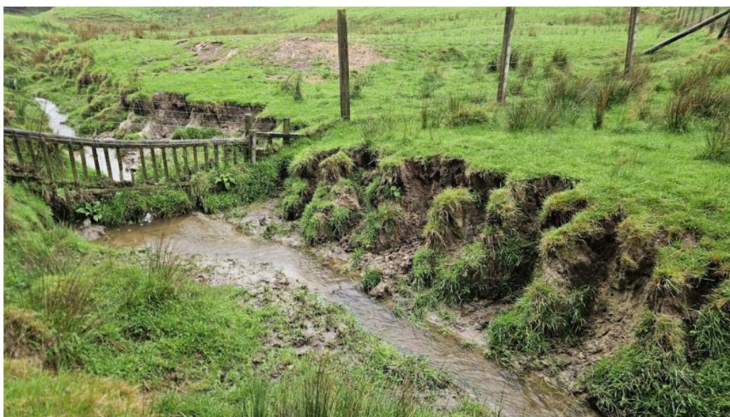
Figure 3. Kakaho Stream tributary, looking upstream to where Retention Wetland E will be located.
