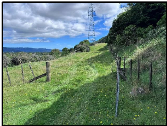
Photo 8: Transmission line on top of land slide debris above the site
