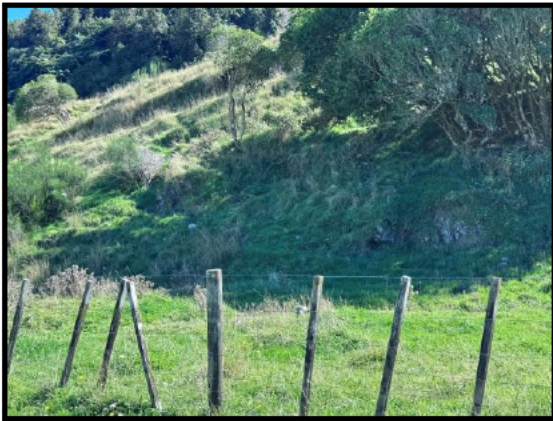
Photo 5: Rock observations where groundwater seepage was observed.
