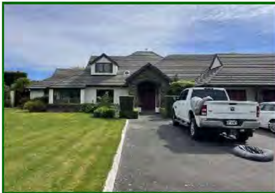
Photo 15 – Dwelling and attached garage
