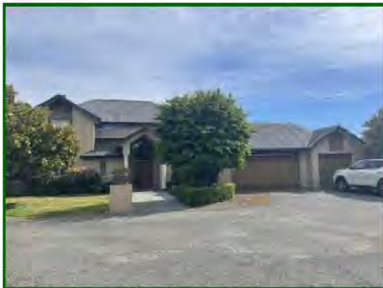
Photo 11 – Dwelling and attached garage
