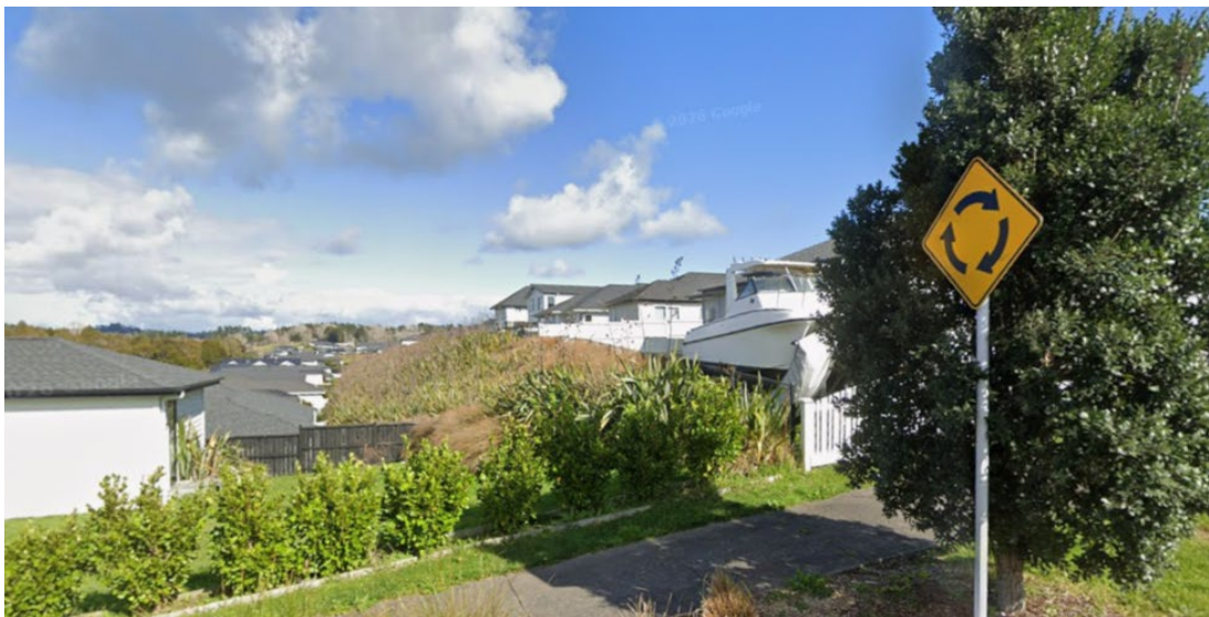
Figure 9 - Existing RE Slope in Milldale (as viewed from Maurice Kelly Road)
