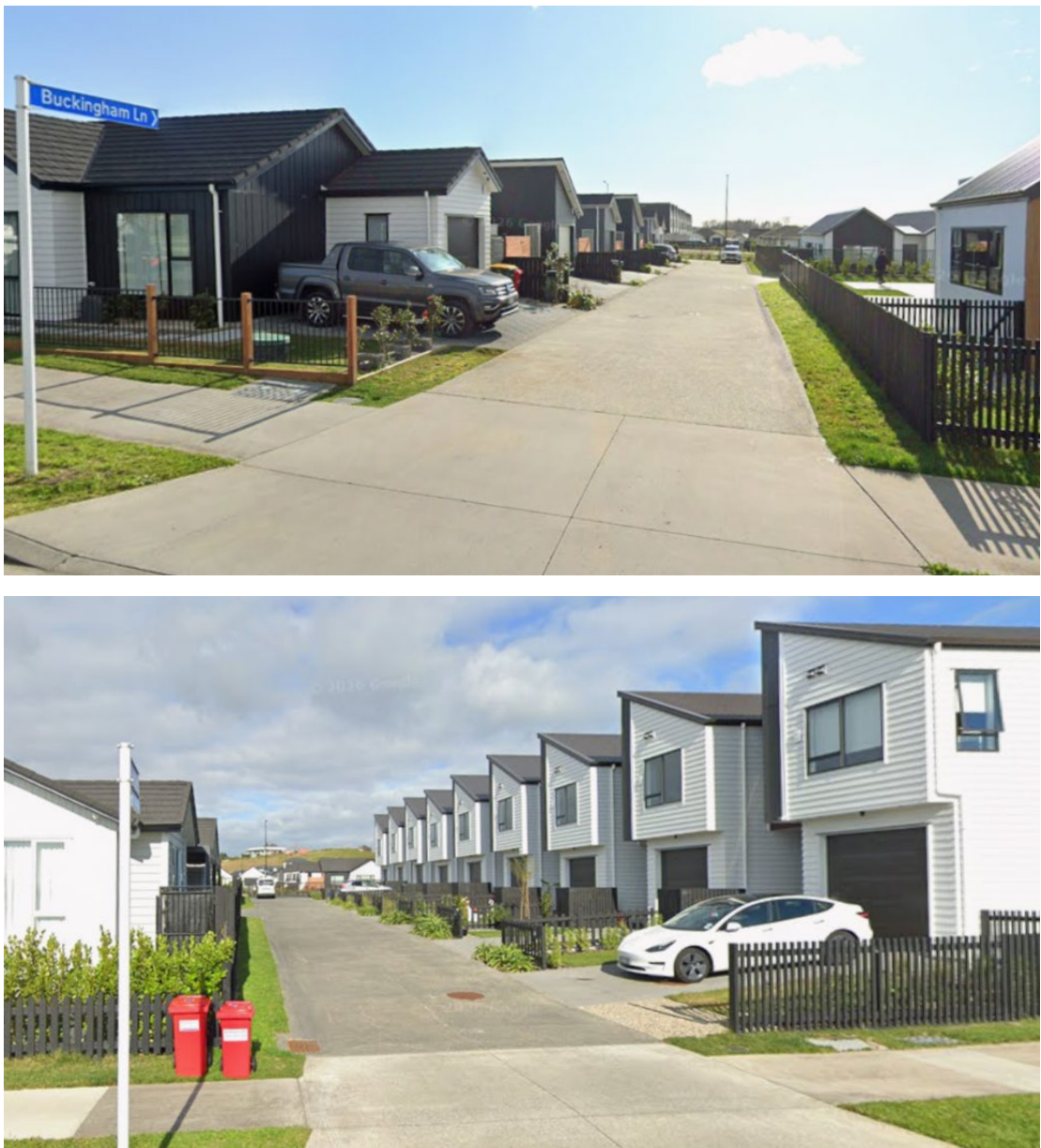
Figure 24 - Existing 7m wide JOALs in Milldale (Buckingham and Emma lanes) (source: Google StreetView)
