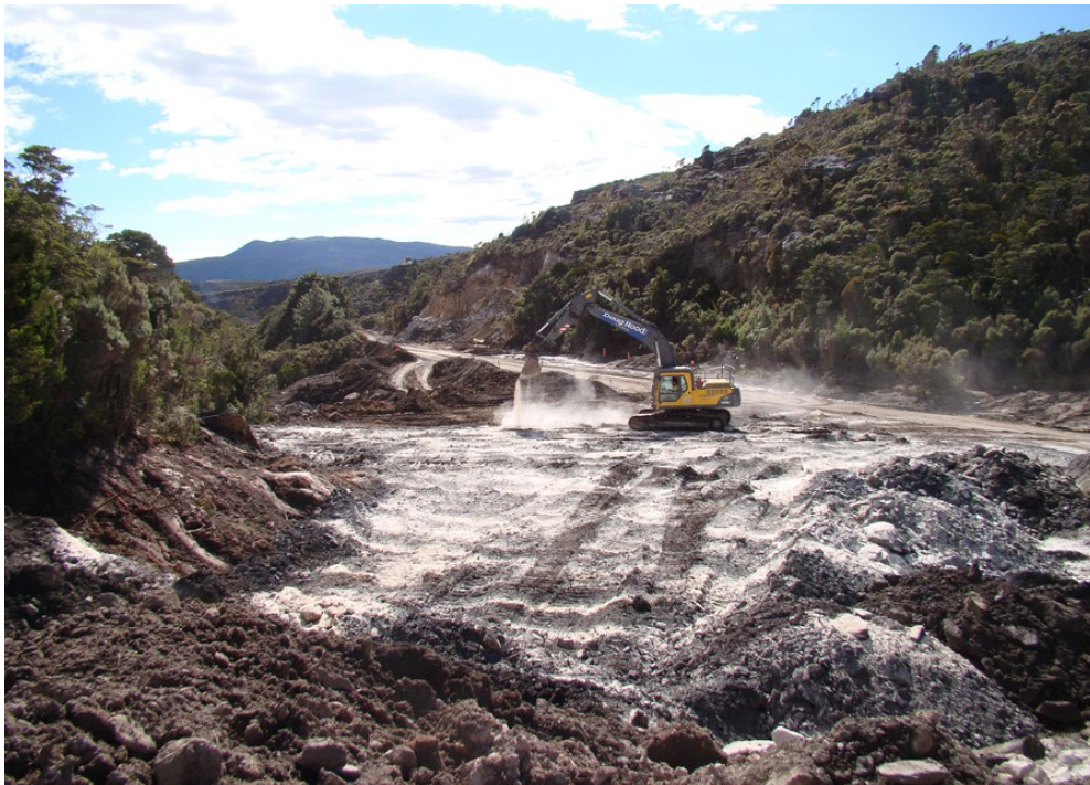
Figure 45. Limestone dosing of the BV ELF.
