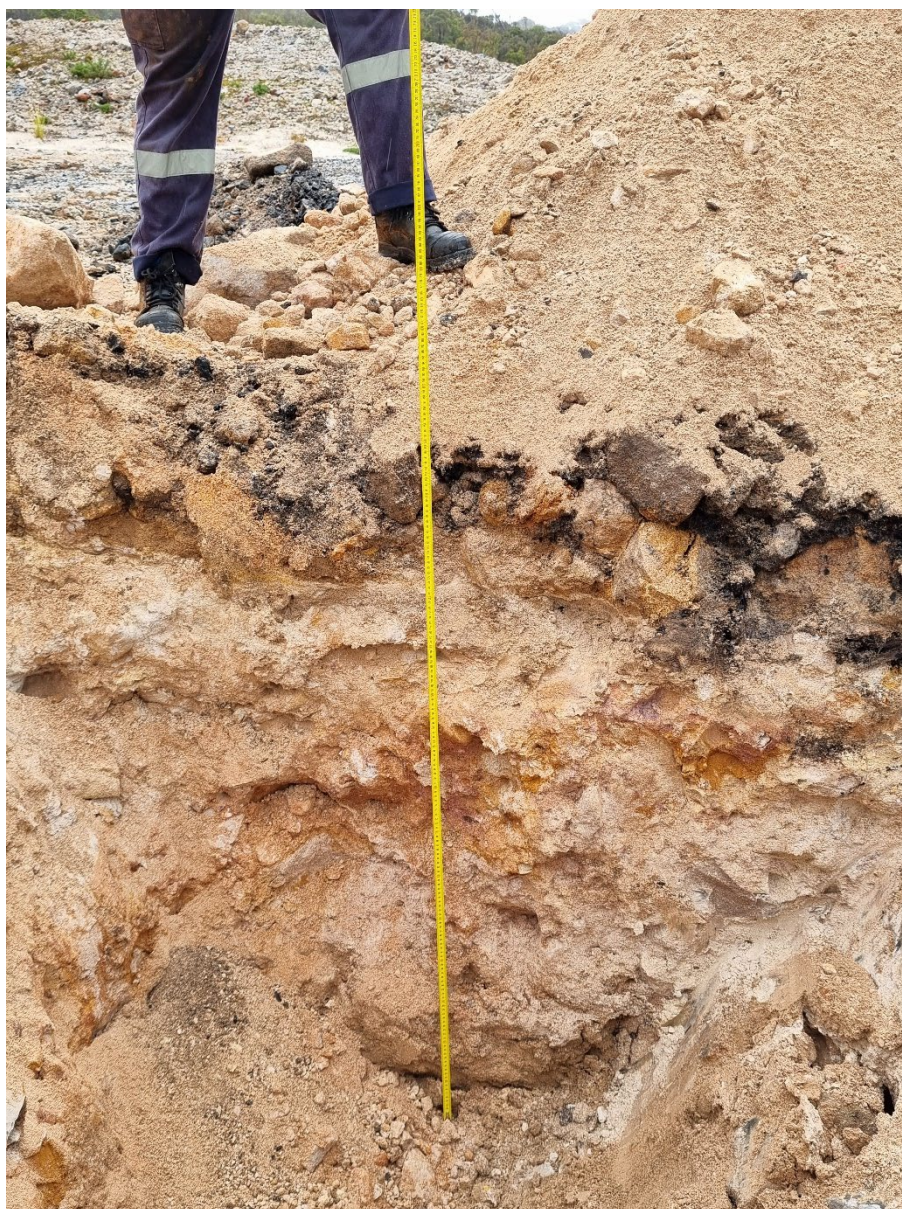
ESC-TP-01: Excavation profiled to 160 cm.
