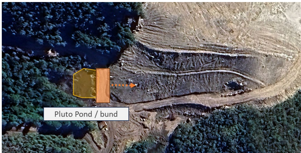
Figure 17: Pluto Pond / Bund and potential seepage to the BV ELF.
