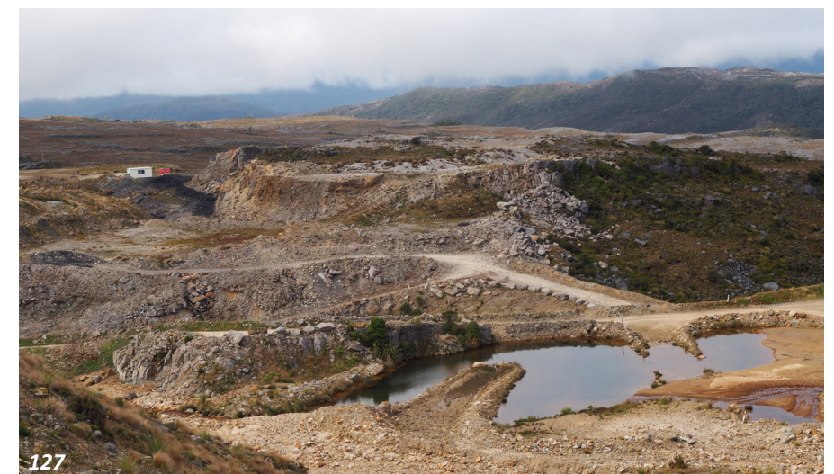
Photograph 125 : Webb Fault escarpment
